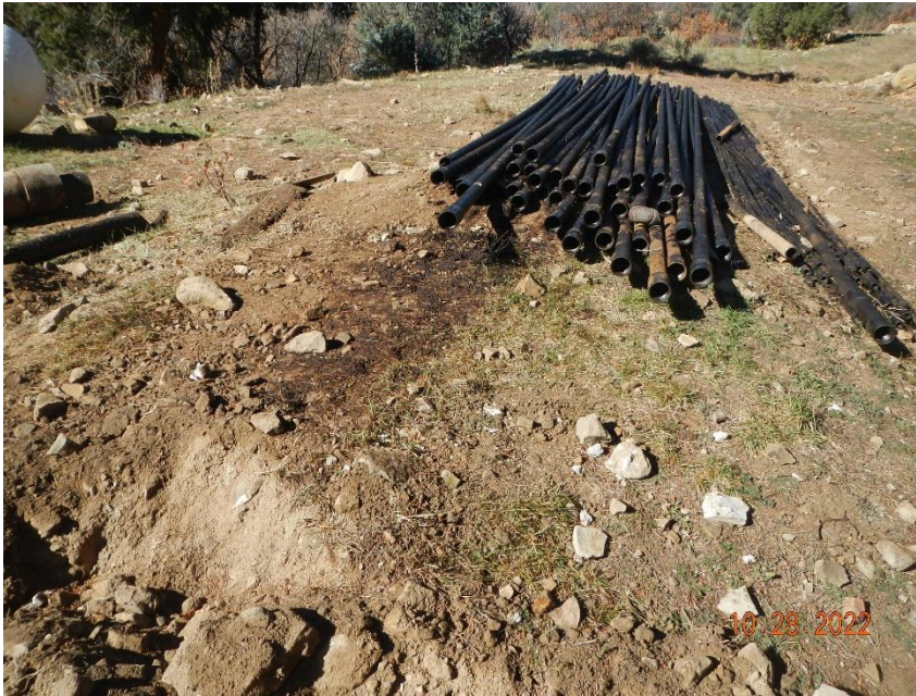
Oily waste on ground, no spill response approx. 18x40"
