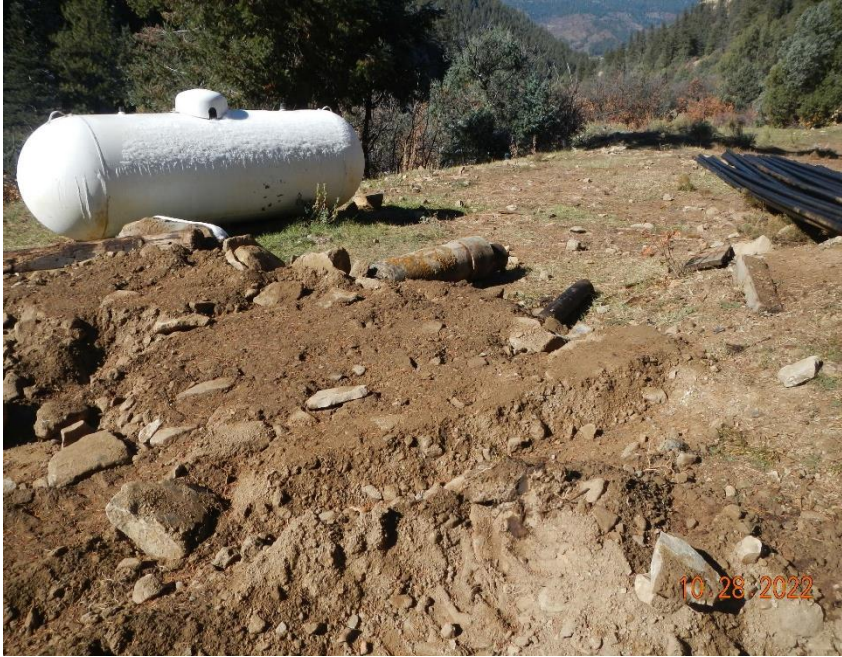
Cut-off stub and backfilled wellhead and propane tank
