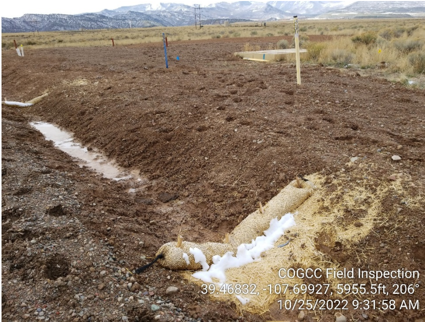
Photo #2 – View of Remediation Project area from north, looking southwest. Note damaged straw wattle in foreground.
