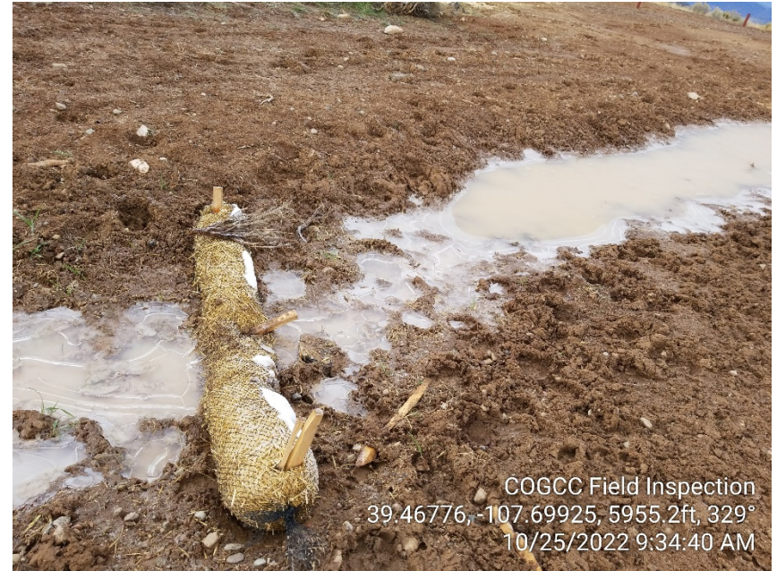
Photo #9 – Straw wattle in roadside ditch located south of Remediation Project area.
