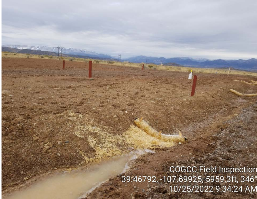
Photo #8 – Four monitoring well risers were observed in Remediation Project area on inspection date. Note damaged straw wattle in foreground.
