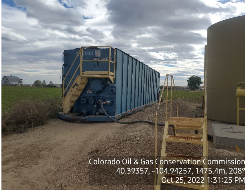
Photo 7: Tank not grounded, no berm surrounding tank
