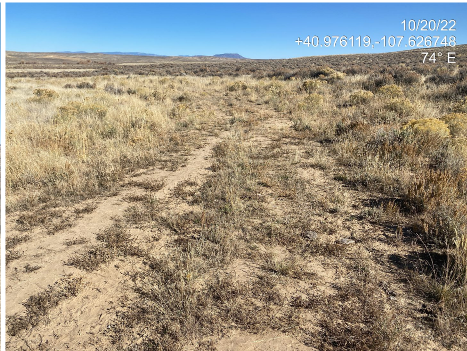
Photo 2. Photo taken to the west of the Location shows the Federal portion of the access road which has been reclaimed. Portions of the road are poorly vegetated. Bare ground and annual weeds are common. Vehicle traffic appears to be impacting reclamation and causing the formation of a two-track.
