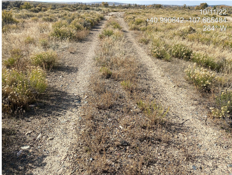
Photo 3. Photo shows a portion of the access road at the southeast. Some areas have soil spread over the top of the pad and road, while others do not. Photo shows the original compacted, graveled access road.
