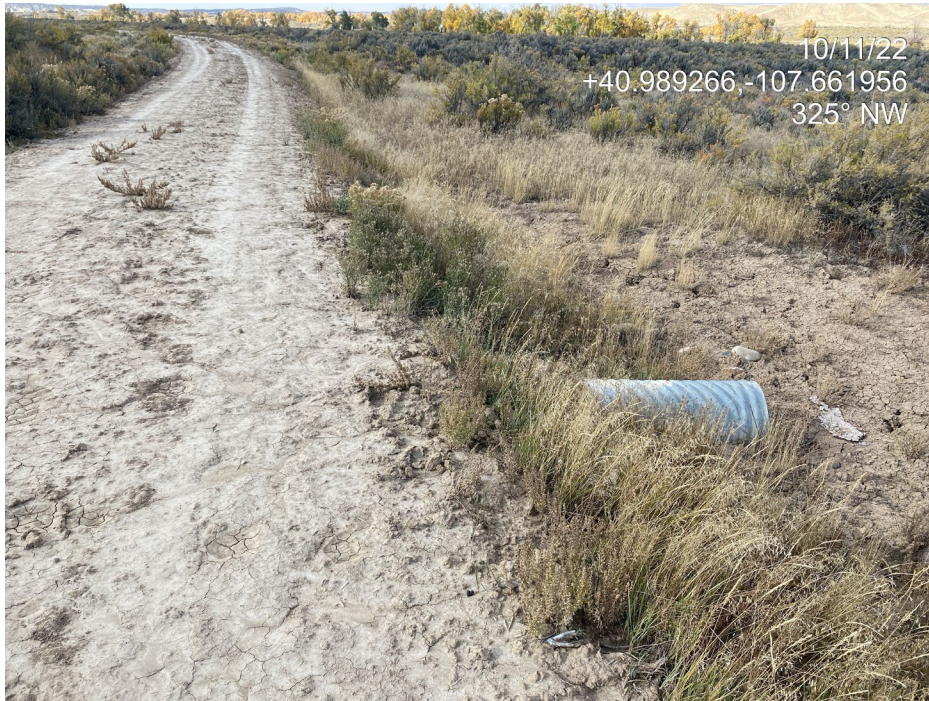
Photo 1. Photo taken to the east shows the access road remains, including multiple culverts. It appears soil has been spread over the top of the original gravel road. Vehicle tracks were evident.
