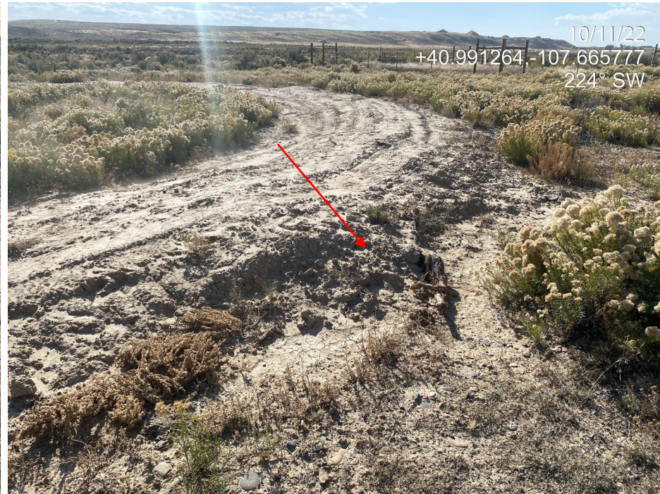
Photo 2. Photo taken from the center of the Location. It appears that road was not properly reclaimed, and that soil was spread over the top of it. The original, compacted, gravel road is evident beneath the soil. Vehicle tracks were evident.
