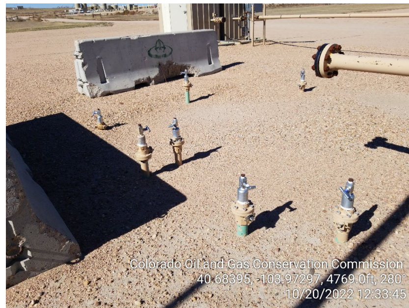
Photo 4 – Unmarked Risers
