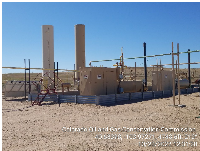
Photo 3 – ECDs and Separators
