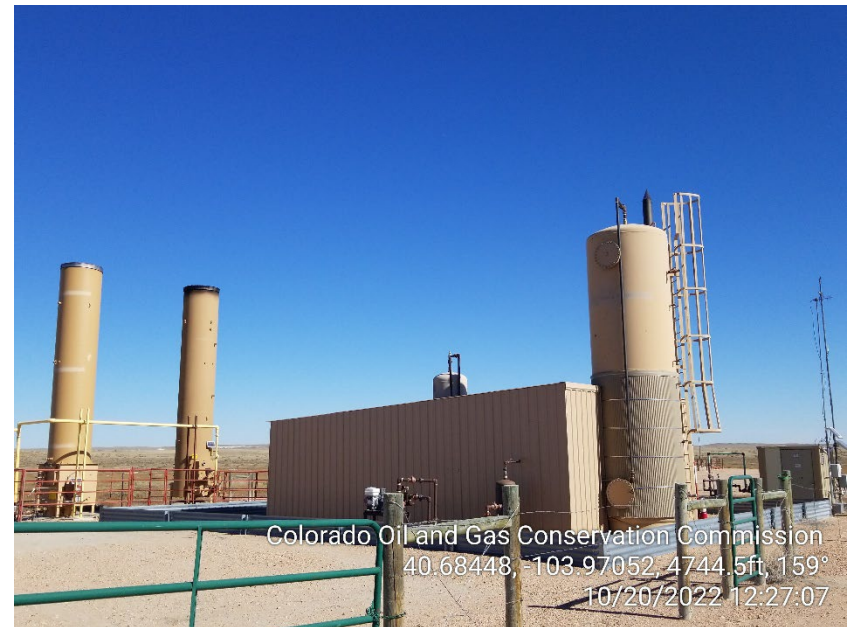
Photo 4 – Heater Treater and ECDs
