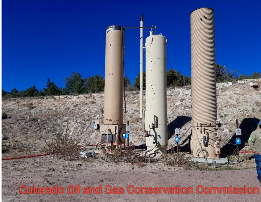
Photo 7 Heated vert sep and ECD's not in use.
