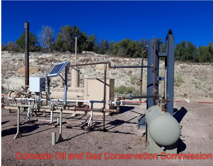
Photo 1 Hoz sep Knock out tanks and meter run
