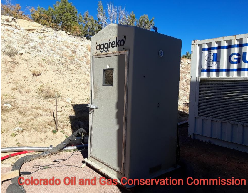
Photo 3 1 of two gas separators for generators
