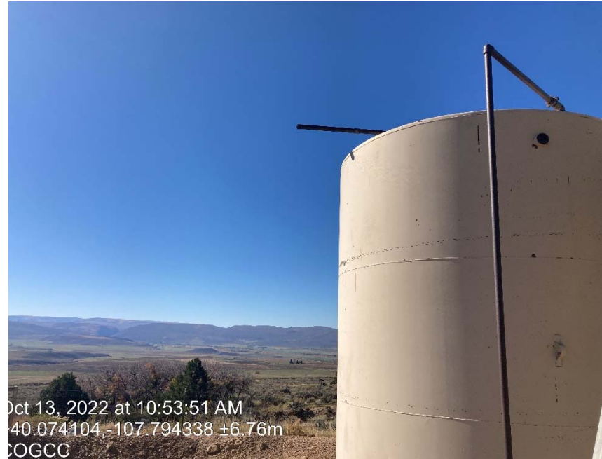
Pipe on top of tank open to atmosphere without a valve or enardo to stop it from venting.
