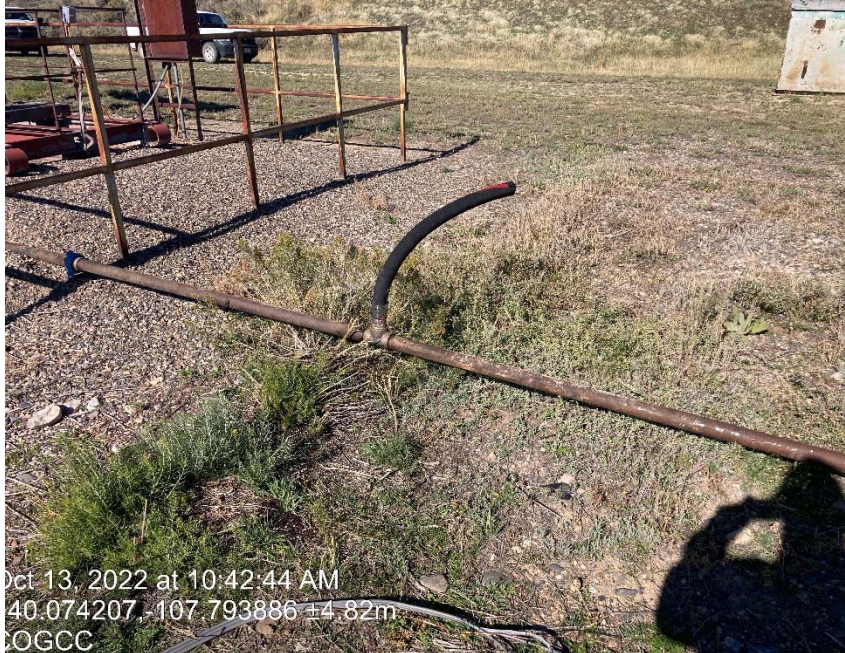
Stored equipment lines are open ended
