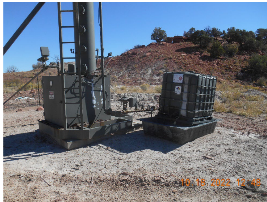
Separator and secondary containment of chemicals
