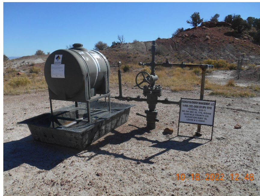
Wellhead with secondary containment of chemicals
