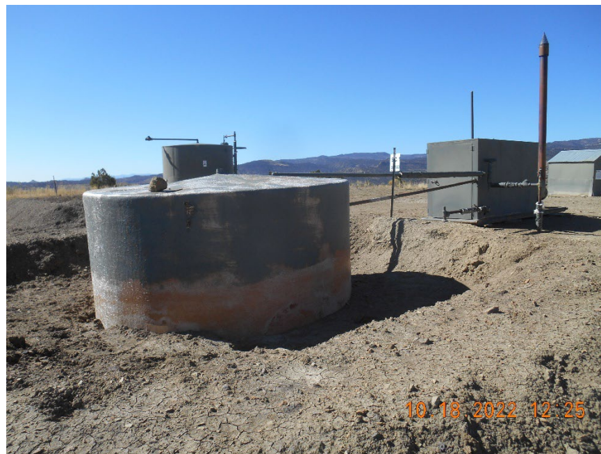
Separator and Produced water tank
