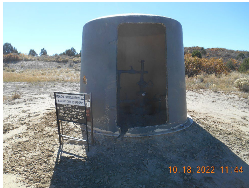
Wellhead inside fiberglass housing
