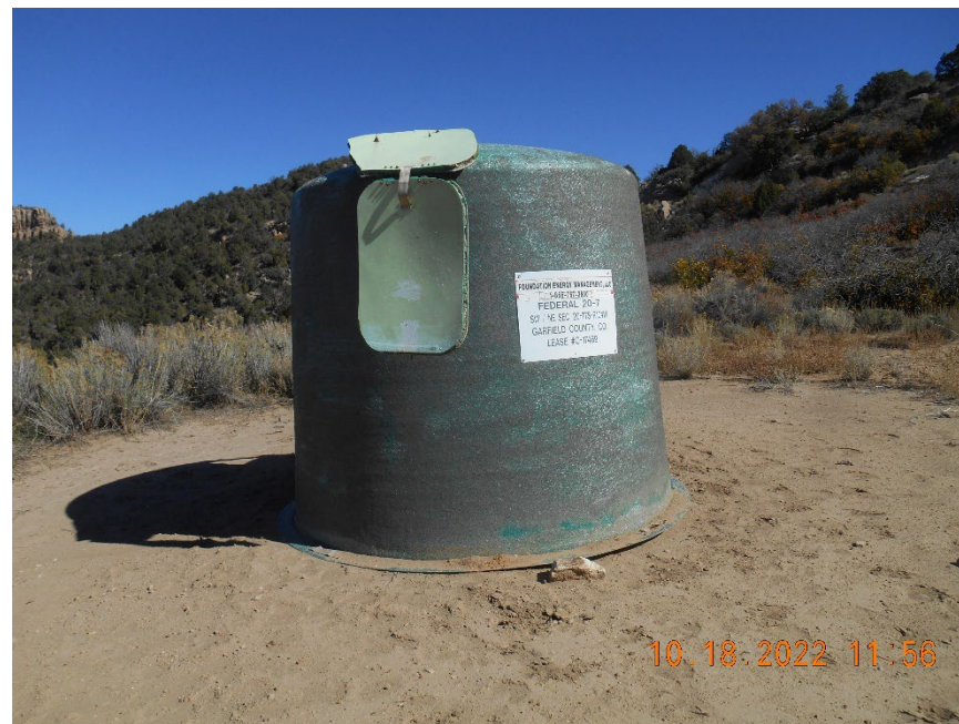
Wellhead inside fiberglass housing
