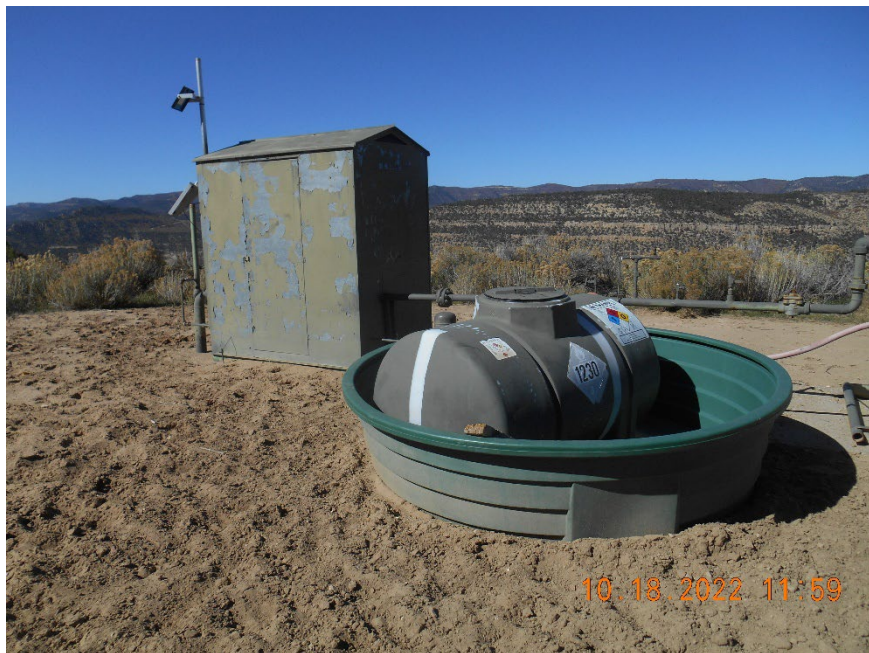
Meter housing and Secondary containment of chemicals
