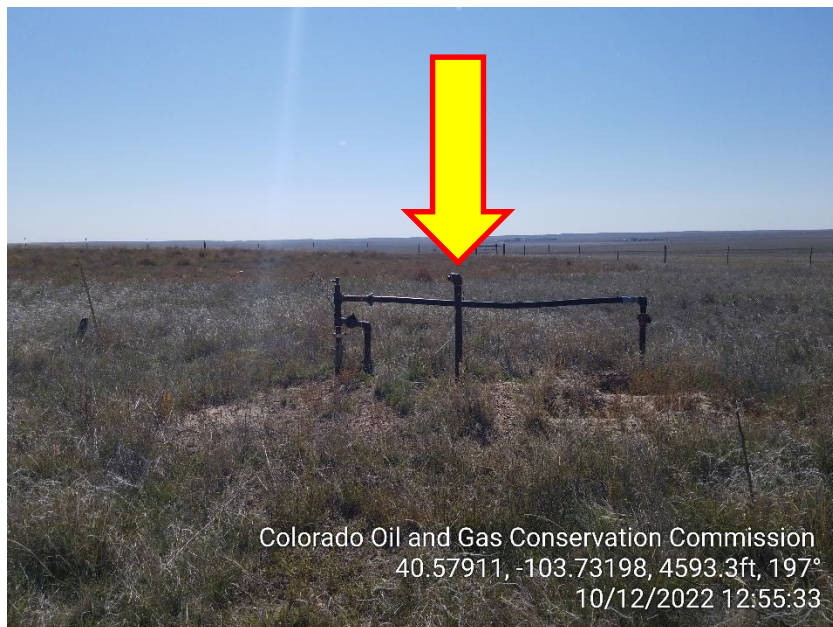
Photo 5 – Unmarked Riser
