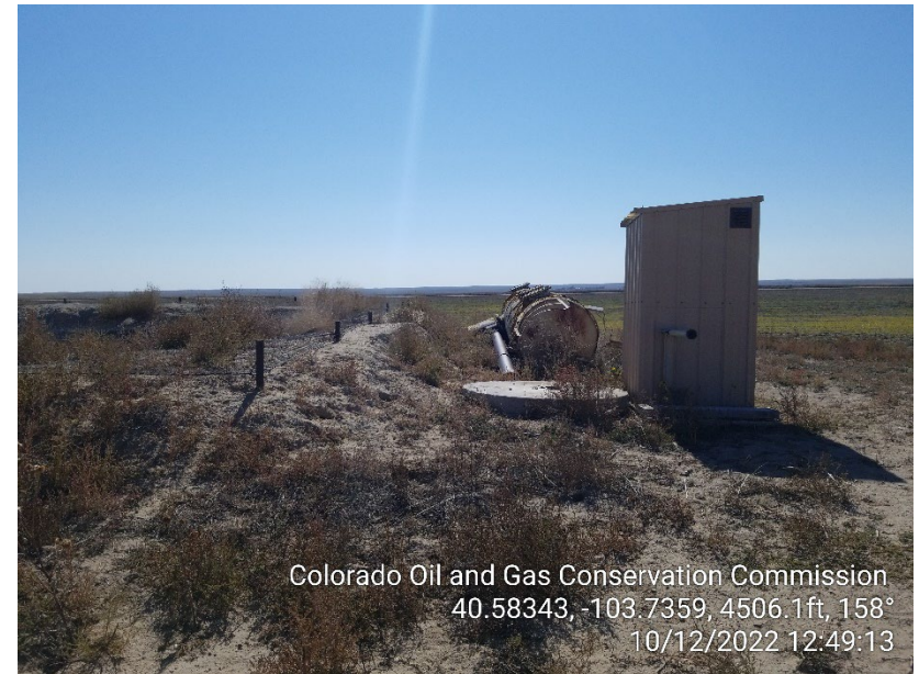
Photo 4 – Unused Heater Treater, Gas Meter Shed and Concrete Pad
