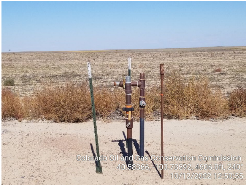
Photo 11 – Unmarked Risers
