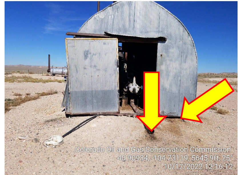
Photo 6 – Gas Engine House – Stained Soil
