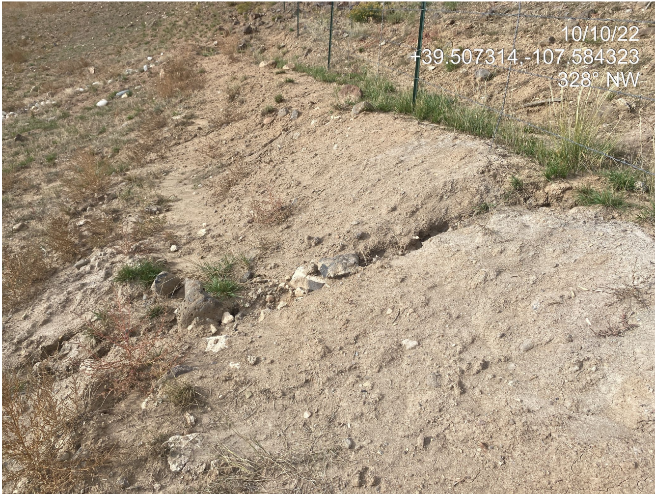
Photo 7. Photo taken from the east shows rill erosion occurring on the eastern slopes of the location.
