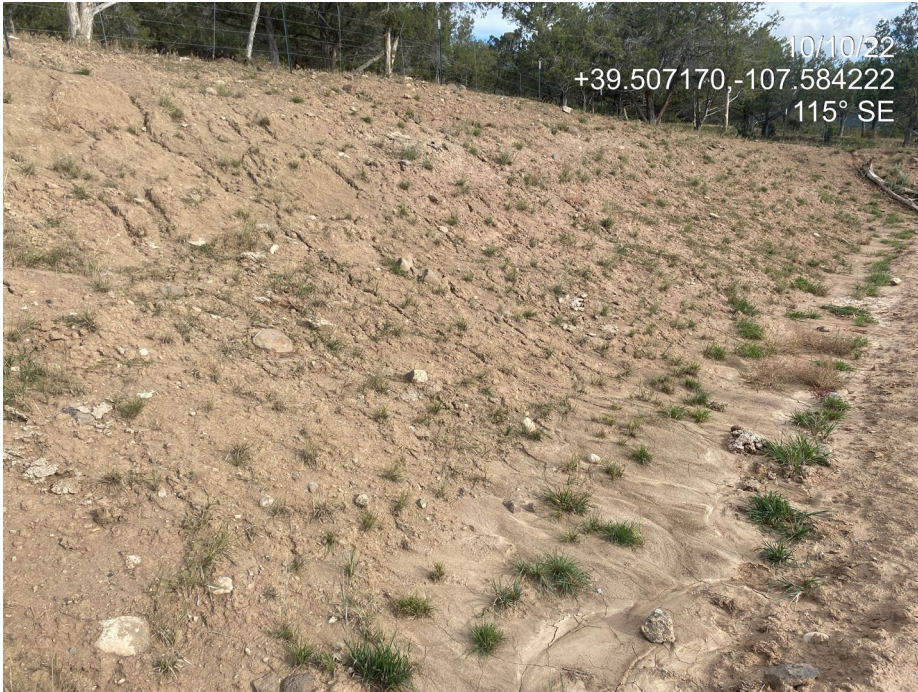
Photo 5. Photo taken from the east shows rill erosion occurring on the eastern slopes of the location.
