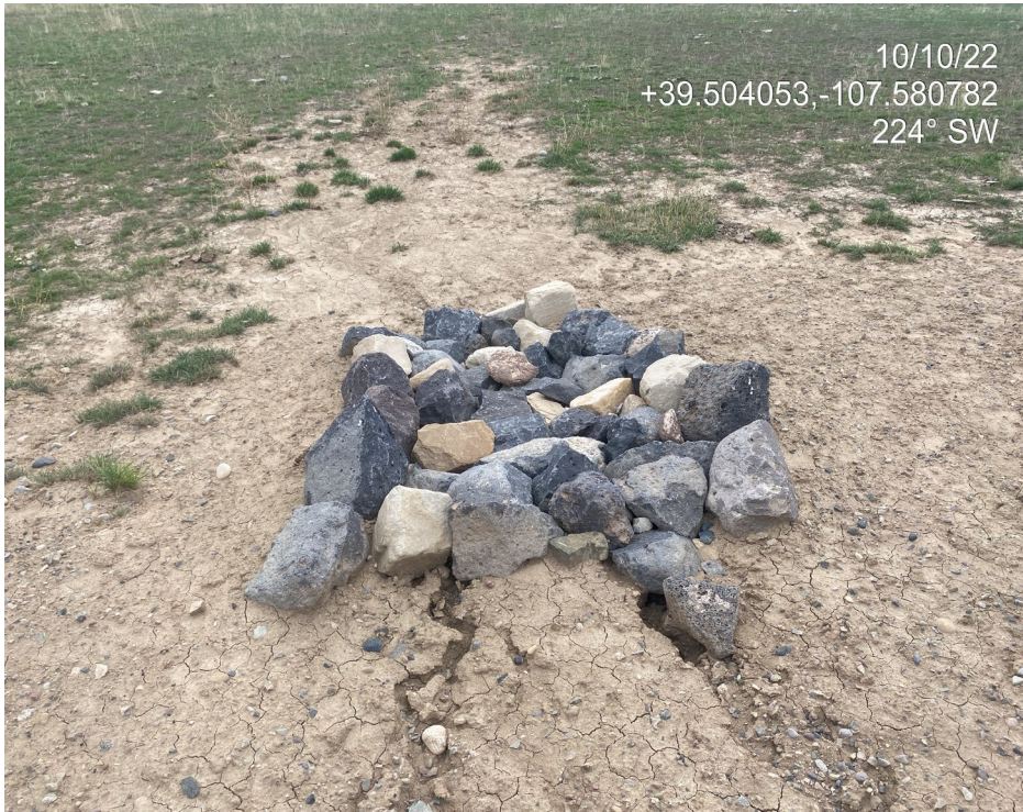
Photo 2. Photo taken to the southwest of the separator shows erosion degradation occurring at a stormwater BMP.
