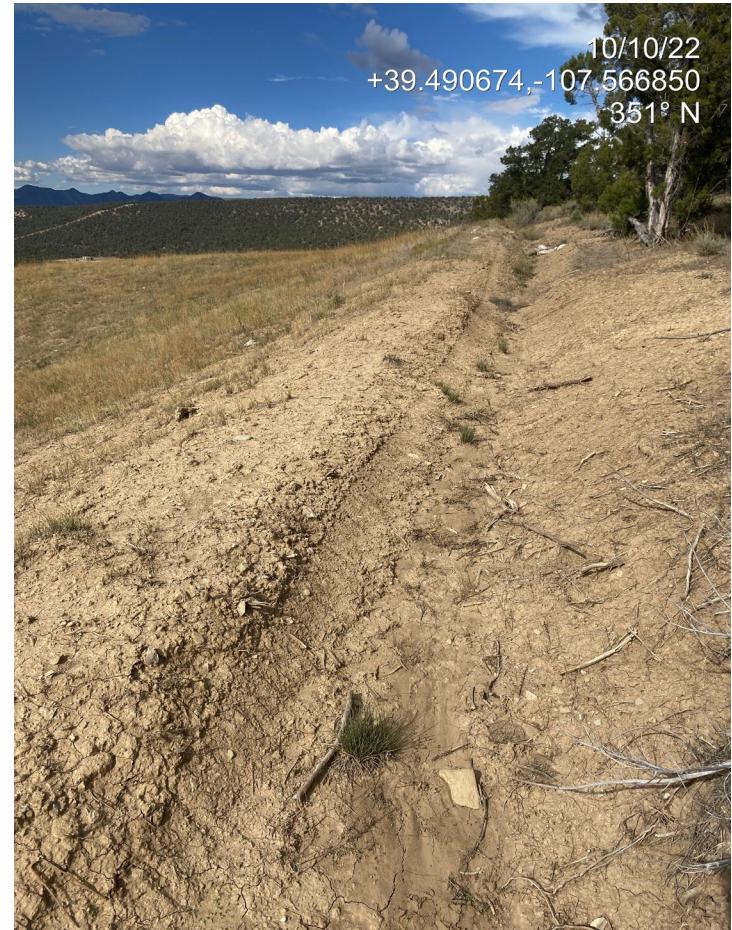
Photo 4. Photo taken from east shows the original cut slope remains, with a stormwater ditch at its base. Contouring will be necessary to address cut slopes/stormwater BMPs during final reclamation.
