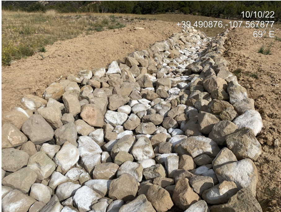
Photo 5. Photo taken from the west shows a slope drain which has been lined with angular riprap and geotextile fabric.
