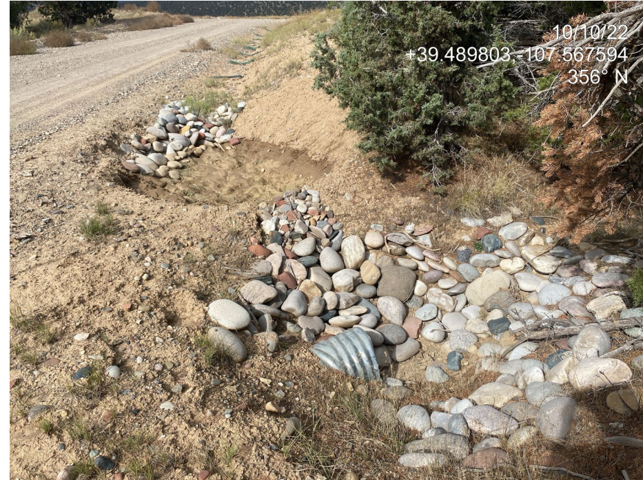
Photo 6. Photo taken from the south shows access road stormwater controls measures.
