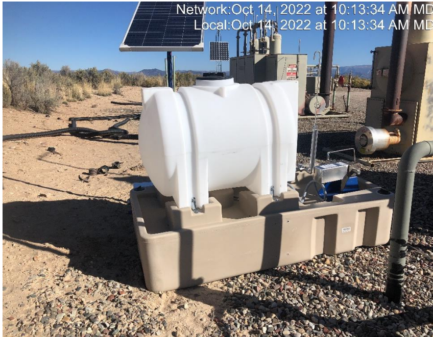
Photo #8068 Chemical tank missing required information.
