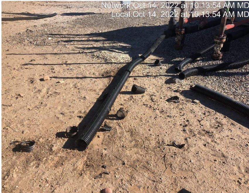
Photo #8070 Multiple heating insulation open ended and not capped.
