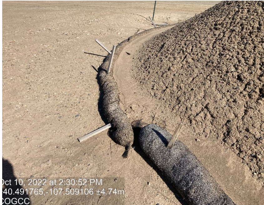
BMP's around dirt pile are failing
