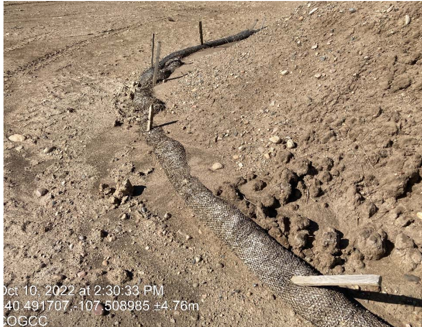
BMP's around dirt pile are failing
