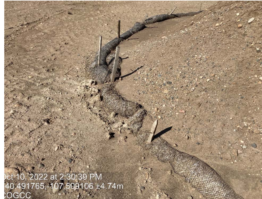
BMP's around dirt pile are failing
