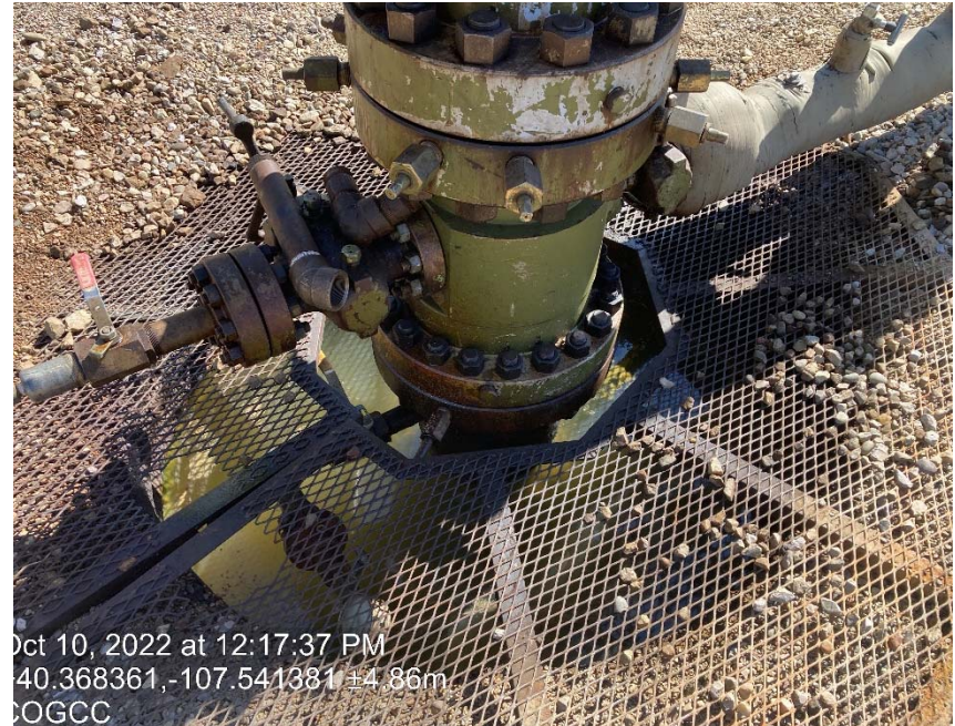
Cellar full of fluid possible hydrocarbons
