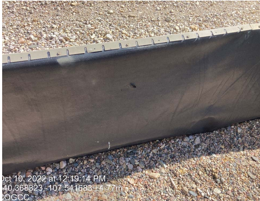
Hole in containment
