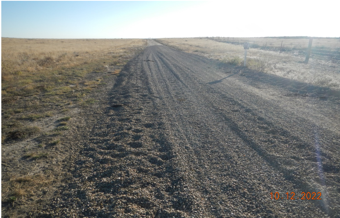
Photo 1. Facing east along the access road. There has been gravel spread along areas of the road. Some areas may have excess gravel that may need to be spread out better.
