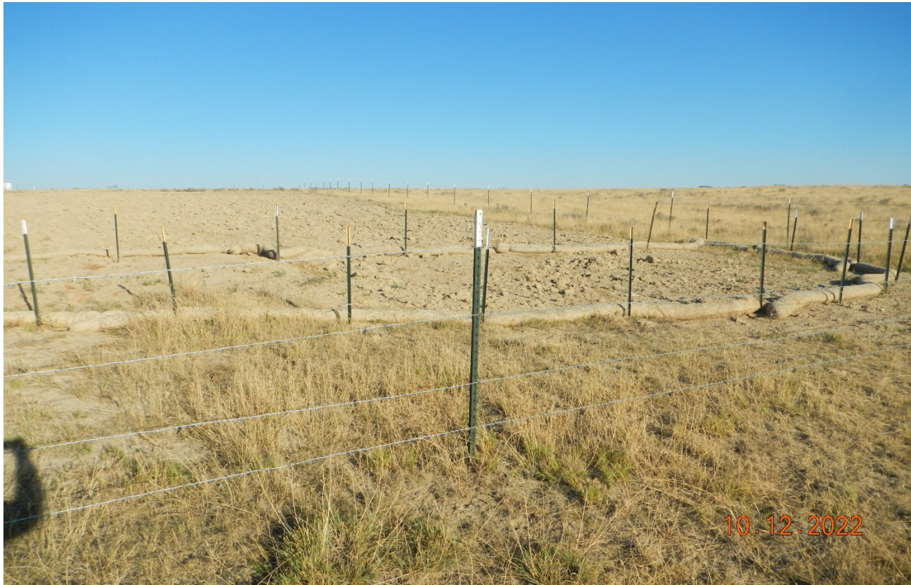
Photo 4. Facing northwest at the location. There are wattles installed at the down gradient side of the location however, wattles are not properly staked down. T-post are being used to hold wattles in place which is not adequate.
