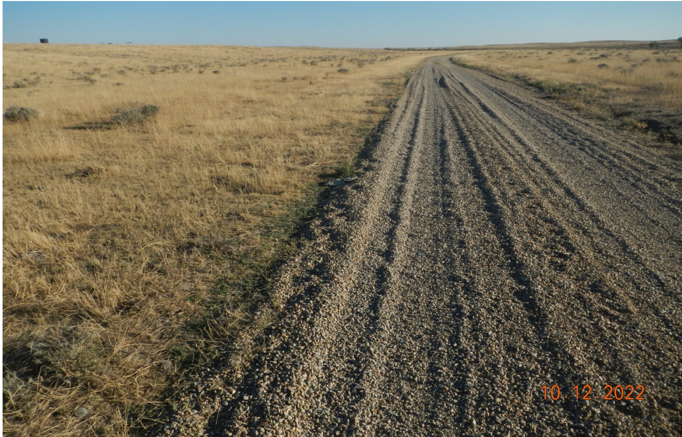
Photo 2. Facing northeast along the access road. There has been gravel spread along areas of the road for stabilization where water was pooling on the road.
