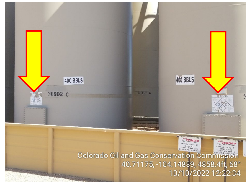
Photo 4 – Labels has faded no longer visible
