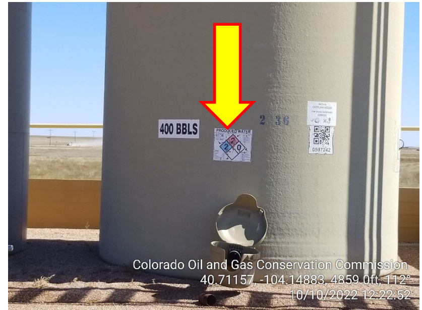
Photo 6 – South Water Tank - Label Fading and peeling away
