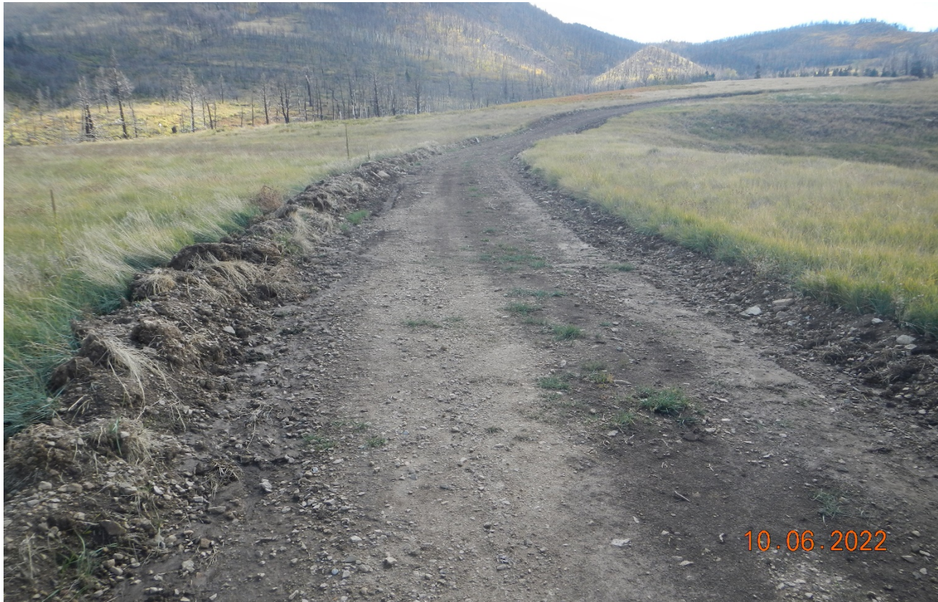
Photo 2. Facing southwest along the access road near the SMU #1-12-B . The road was graded along a portion of the road. The concern now is lack of BMP's on this long stretch or road which will direct stormwater and create more erosion.
