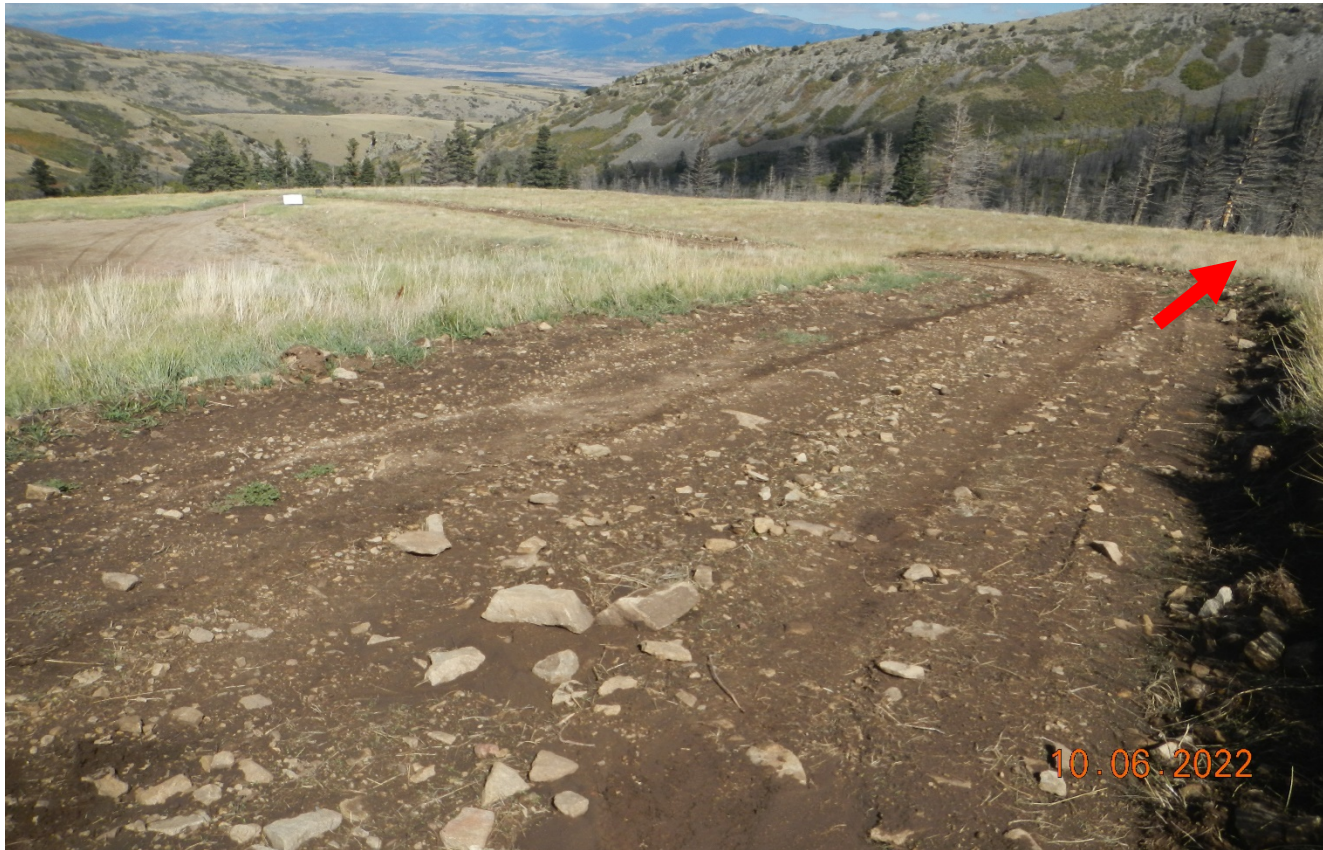
Photo 3. Facing northeast. The road will direct stormwater all the way down the road creating erosion. BMP's need to be installed to direct stormwater off the road and reduce stormwater concentration along the road. A diversion ditch would be helpful at the red arrow along with water bars, sediment traps, check dams, ect.
