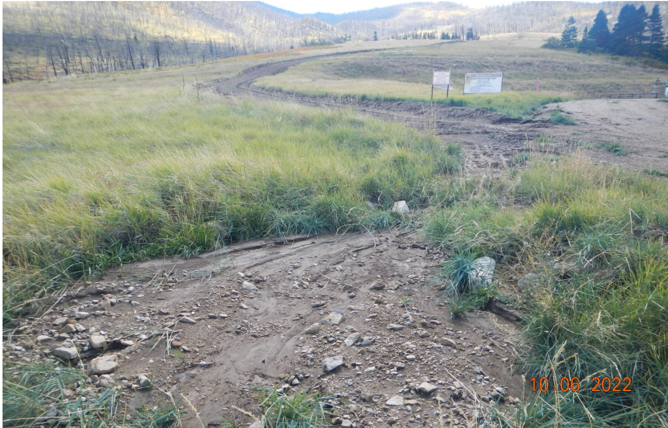
Photo 1. Facing southwest along the access road near the SMU #1-12-B . There is sediment from the road depositing in this area. BMP's such as a sediment trap should be installed in this area.
