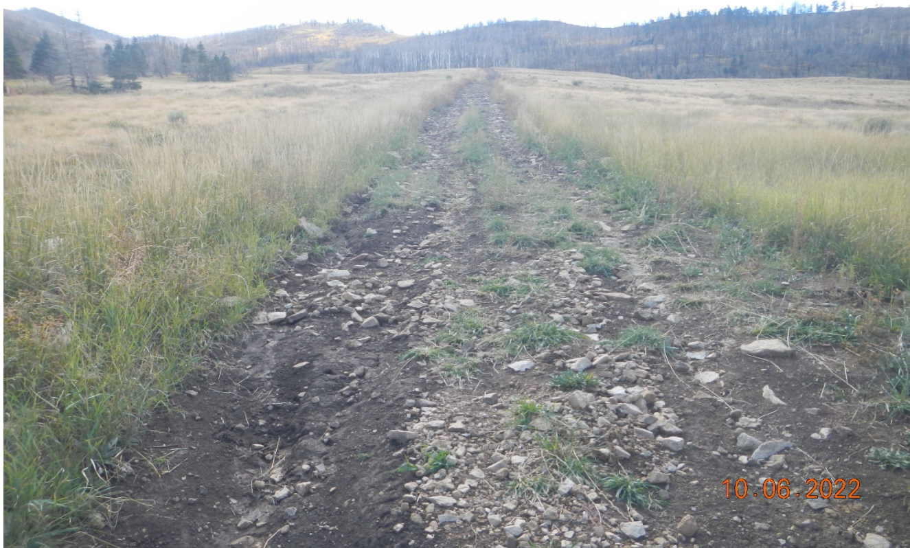
Photo 5. Facing southwest. The grading ended at this point which appears to be more stabilized with vegetation. Did not inspect any further due to wet soil conditions.
