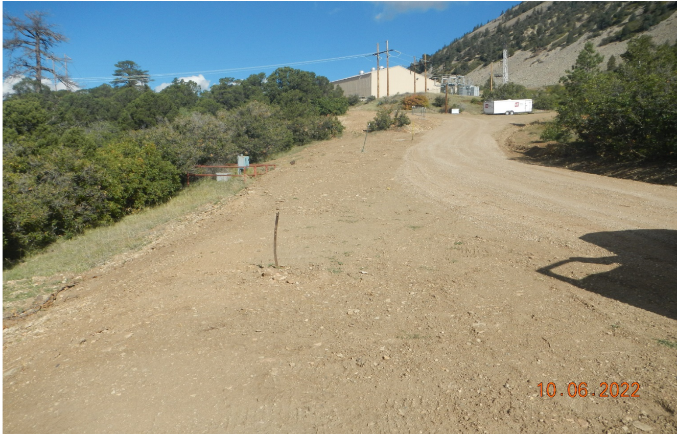
Photo 1. Facing north along the access road. The disturbance from the flowline along the road needs to be reclaimed and stabilized.
