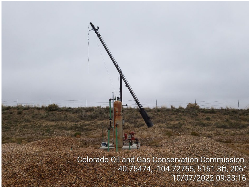
Photo 7 – Flare – Disconnected
