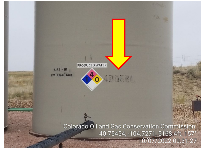
Photo 4 – Label has faded no longer visible
