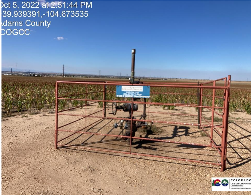
Pic 1 wellhead
