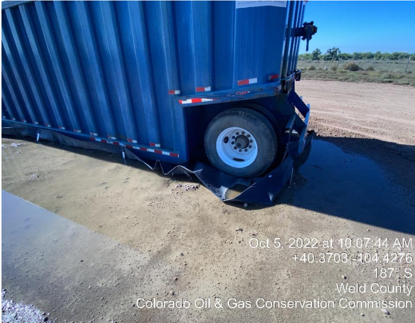
Photo #3 Inadequate Berms
