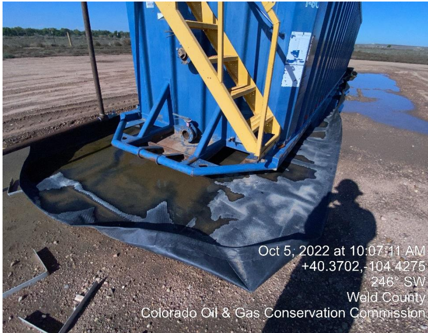
Photo #1 Inadequate Berms
