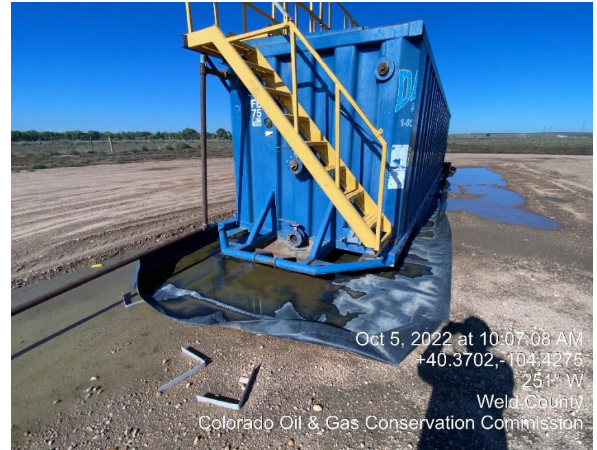
Photo #2 Inadequate Berms
