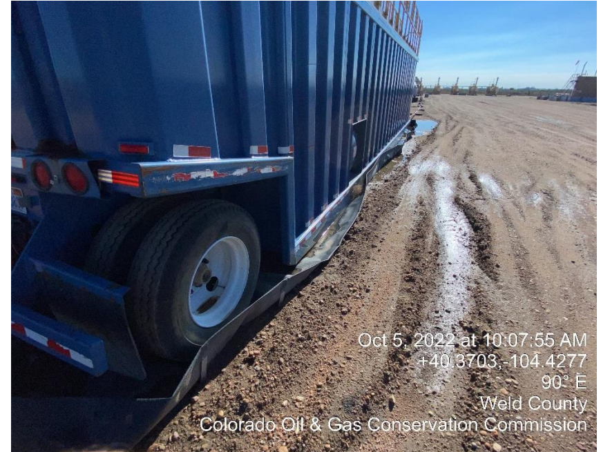
Photo #4 Inadequate Berms
