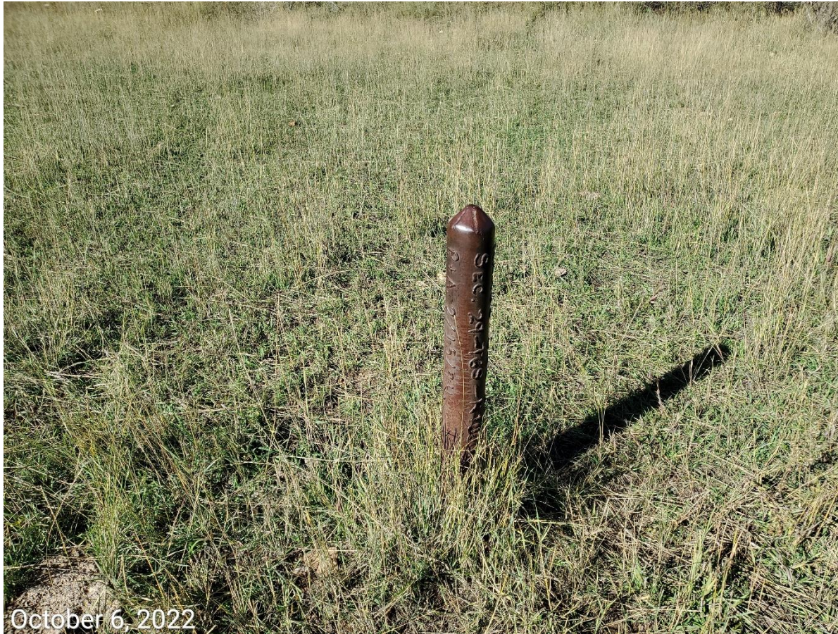
Photo 3: Photo shows well marker for the DA Federal 23-29 well, plugged by North American Resources Company
