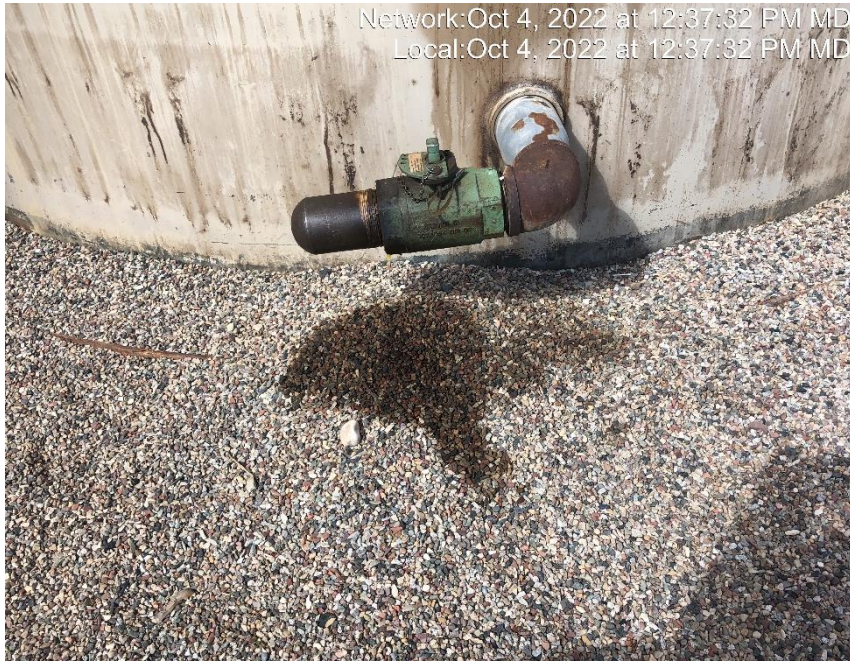
Photo #7923 Stained soils in containment.
