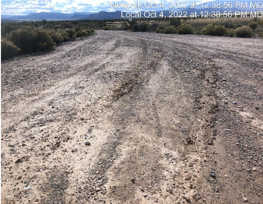
Photo #7925 Insufficient tracking BMP at entrance to location.
