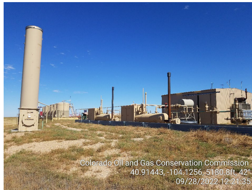
Photo 4 – ECD and Separators
