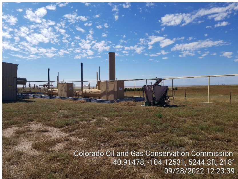
Photo 9 – Separators and VRU
