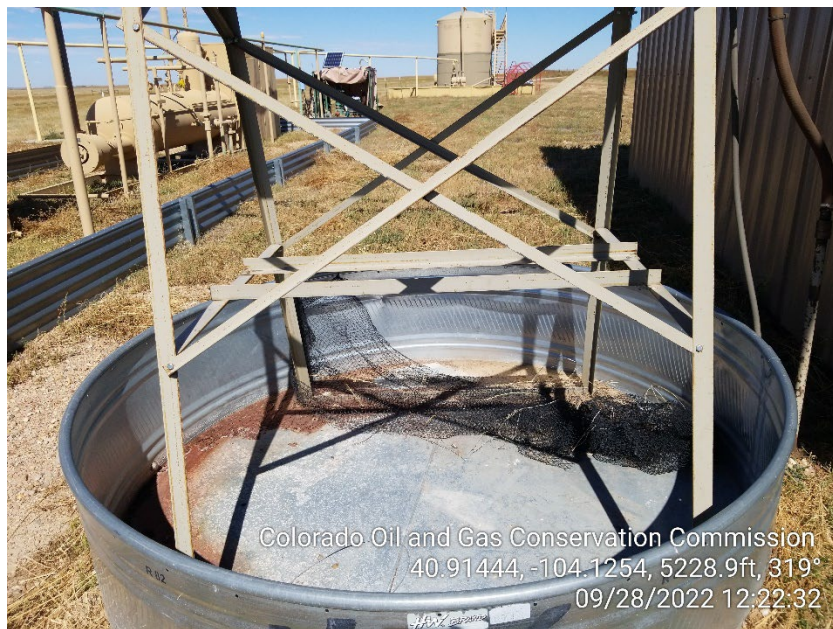
Photo 7 – Day Tank Wildlife Netting in disrepair
