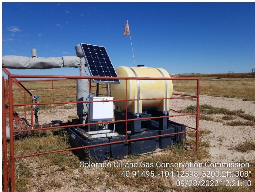
Photo 3 – Chemical Tank missing Labels
