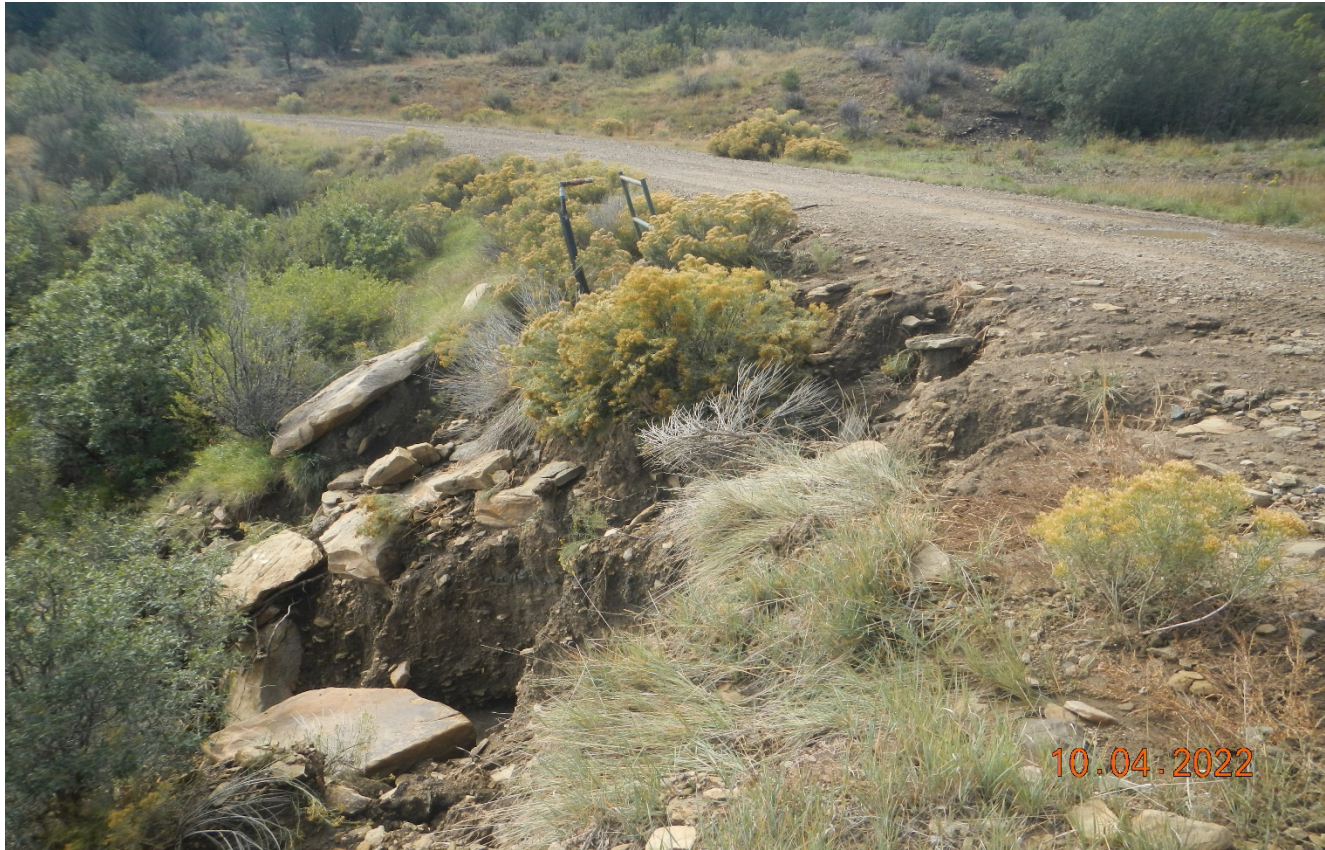
Photo 1. Facing south along the access road. There is significant erosion occurring across the road in this area. This area has no culvert and stormwater from the drainage washes across the road. Lat/Long:37.10005,-104.76045
