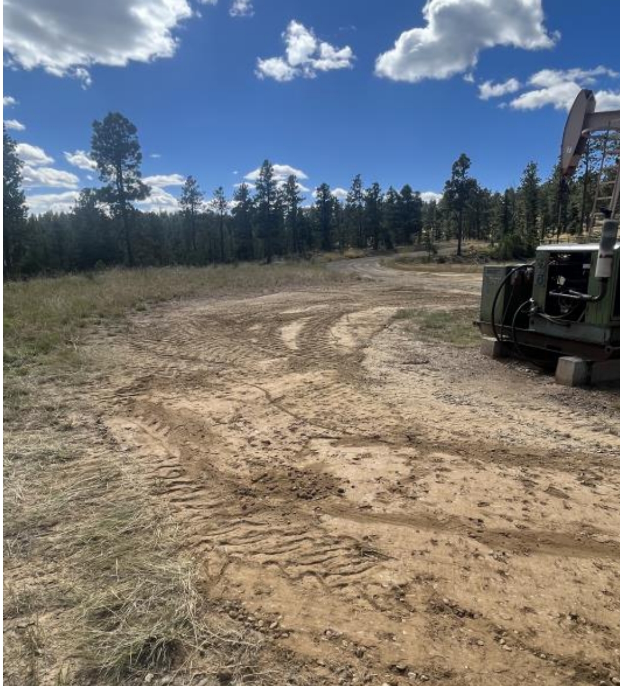
PHOTO 1: THE LEAKING PACKING BOLT HAS BEEN TIGHTENED AND MAINTENANCE HAS BEEN PERFORMED TO ENSURE ALL VALVES, PIPES, FITTINGS ARE SECURELY FASTENED. ALL PRODUCTION EQUIPMENT ARE IN GOOD MECHANICAL CONDITION. THE WELL PAD HAS BEEN BLADED AND GROOMED TO ELIMINATE THE VEHICLE RUTTING. DIVERSION DITCHES ALONG THE ACCESS LEADING TO THE LOCATION HAVE BEEN REDEFINED TO BETTER DIRECT STORMWATER OFF OF LOCATION.
