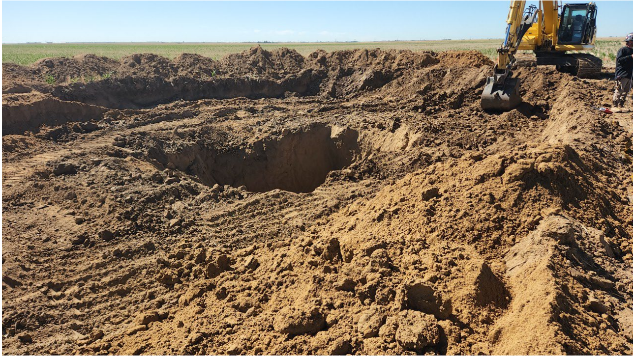
#1A – Champlin 67F – Excavation Overview – Facing SE – Outer 3ft SAR Exceedance Excavation – Inner 15ft Petroleum Exceedance Excavation
