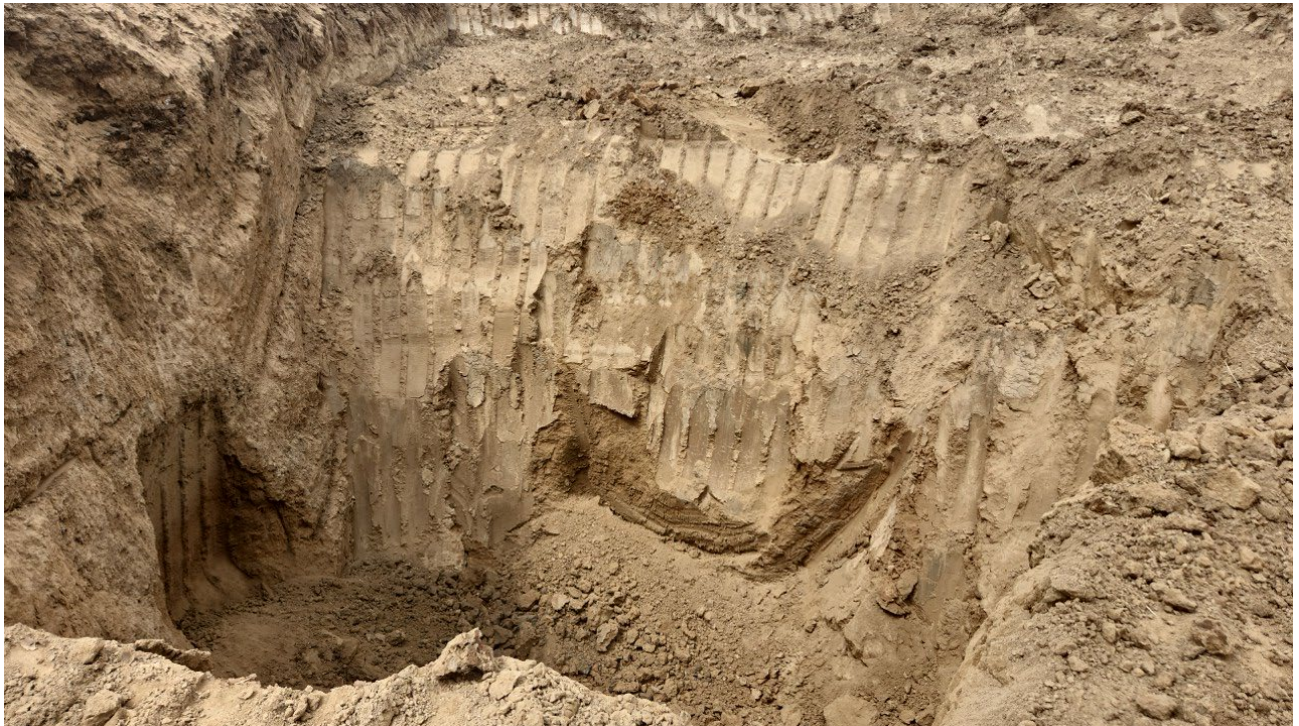
#4A – Champlin 67F – Inner Petroleum Exceedance Excavation – Former Produced Water Pit – Northern Sidewall of Excavation – N01@12.0' – PID 0.0ppm – Sample Submitted for Lab Analysis
