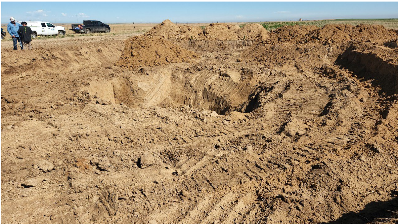
#2A – Champlin 67F – Excavation Overview – Facing NW – Outer 3ft SAR Exceedance Excavation – Inner 15ft Petroleum Exceedance Excavation
