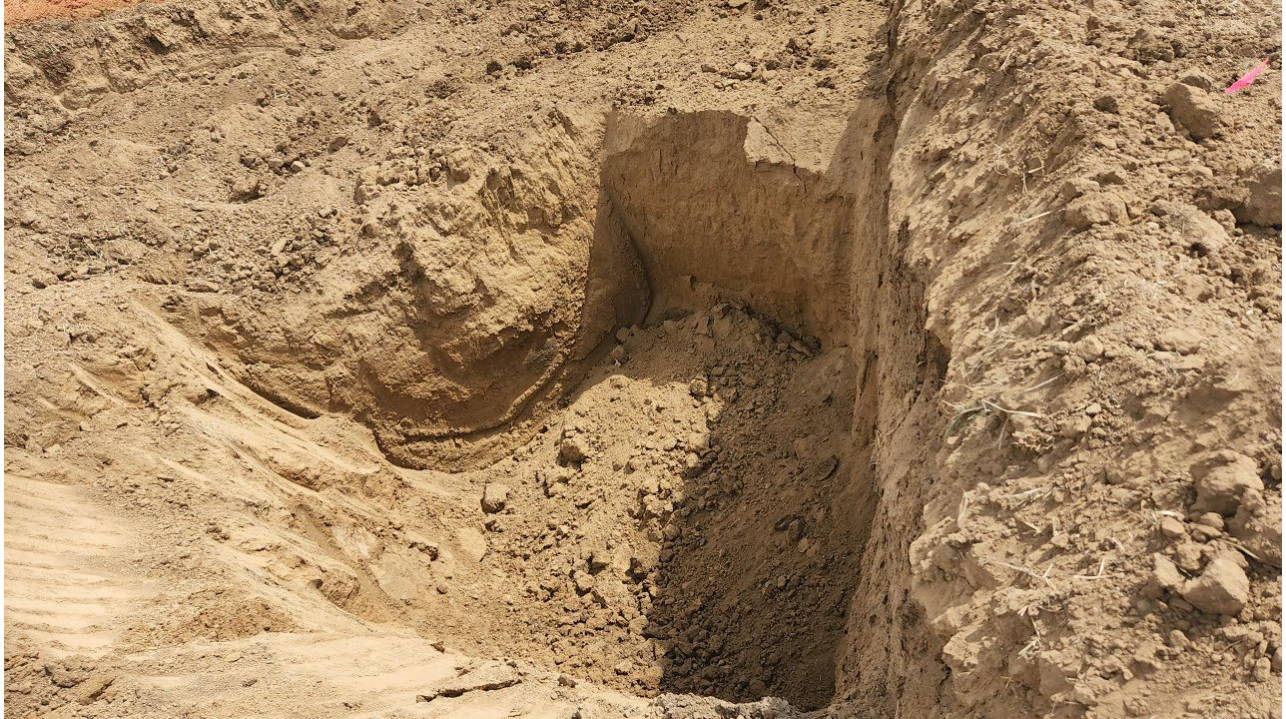
#3A – Champlin 67F – Inner Petroleum Exceedance Excavation – Former Produced Water Pit – Base of Excavation – B01@15.0' – PID 4.2ppm – Sample Submitted for Lab Analysis
