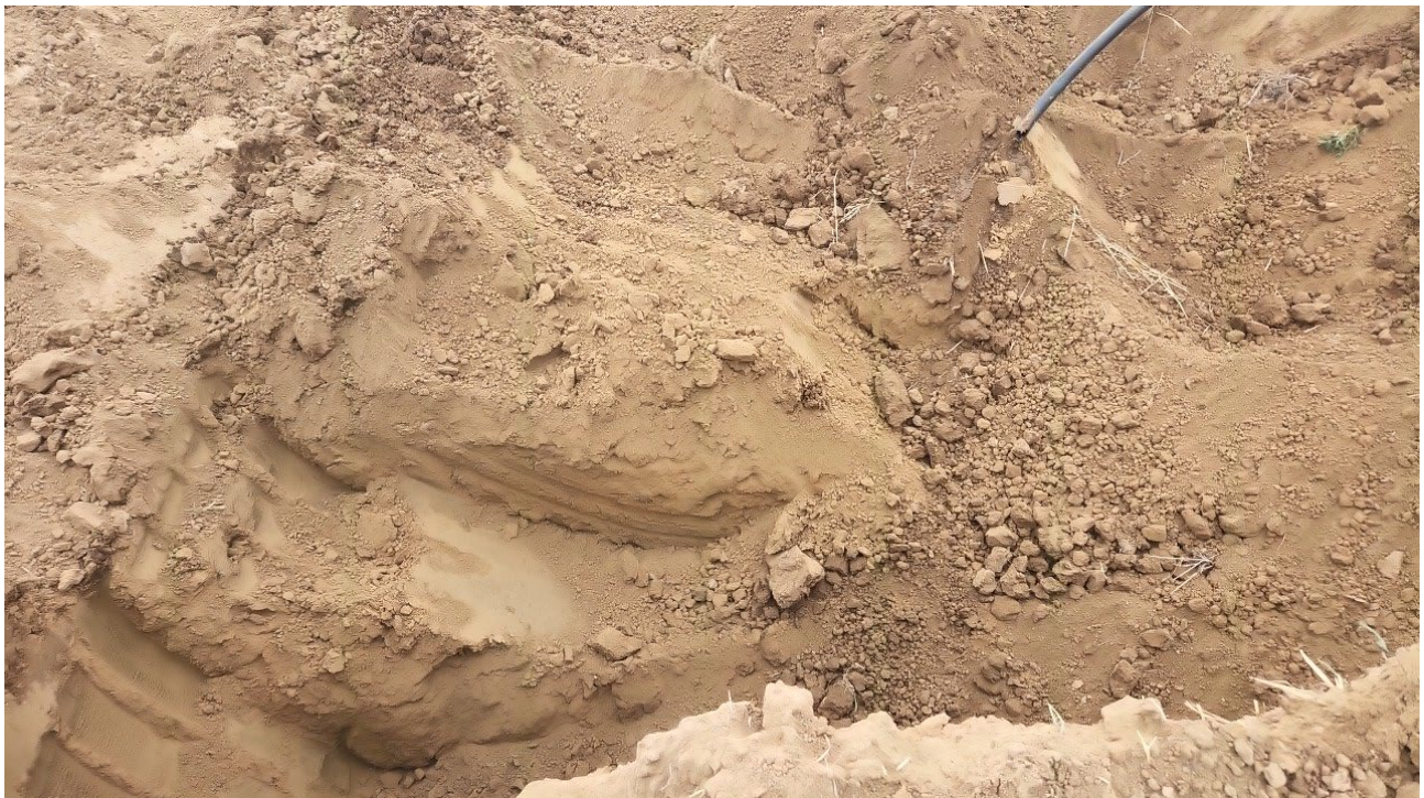
#6A – Champlin 67F – Inner Petroleum Exceedance Excavation – Former Produced Water Pit – Eastern Sidewall of Excavation – E01@10.0' – PID 1.4ppm – Sample Submitted for Lab Analysis
