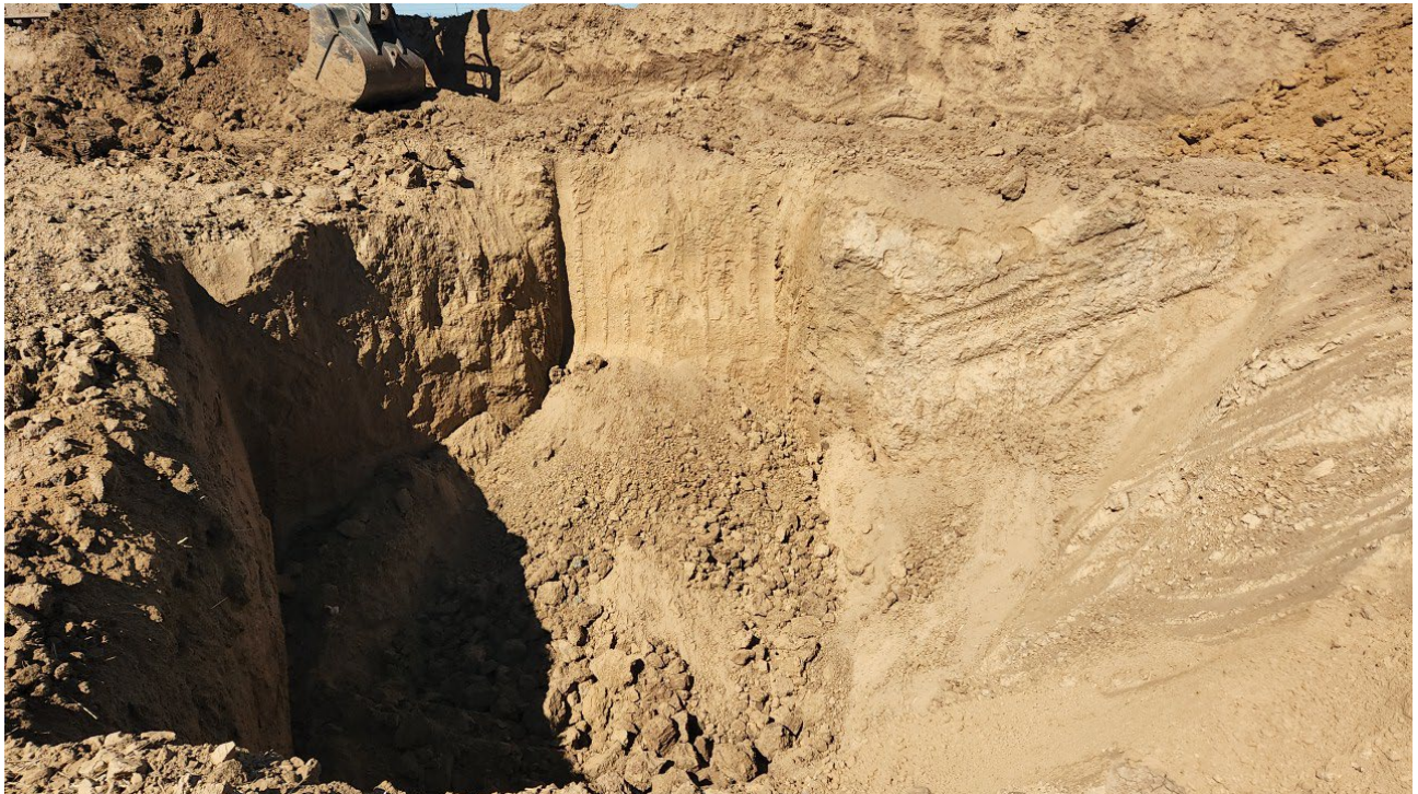
#8A – Champlin 67F – Inner Petroleum Exceedance Excavation – Former Produced Water Pit – Second Sample of Western Sidewall – W02@12.0' – PID 0.0ppm – Sample Submitted for Lab Analysis
