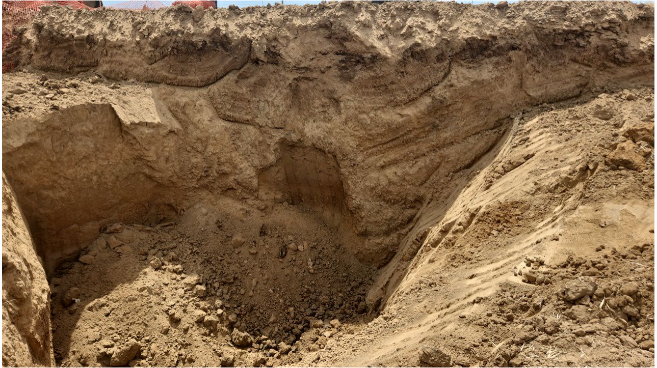
#7A – Champlin 67F – Inner Petroleum Exceedance Excavation – Former Produced Water Pit – First Sample of Western Sidewall – W01@12.0' – PID 10.4ppm – Sample Submitted for Lab Analysis
