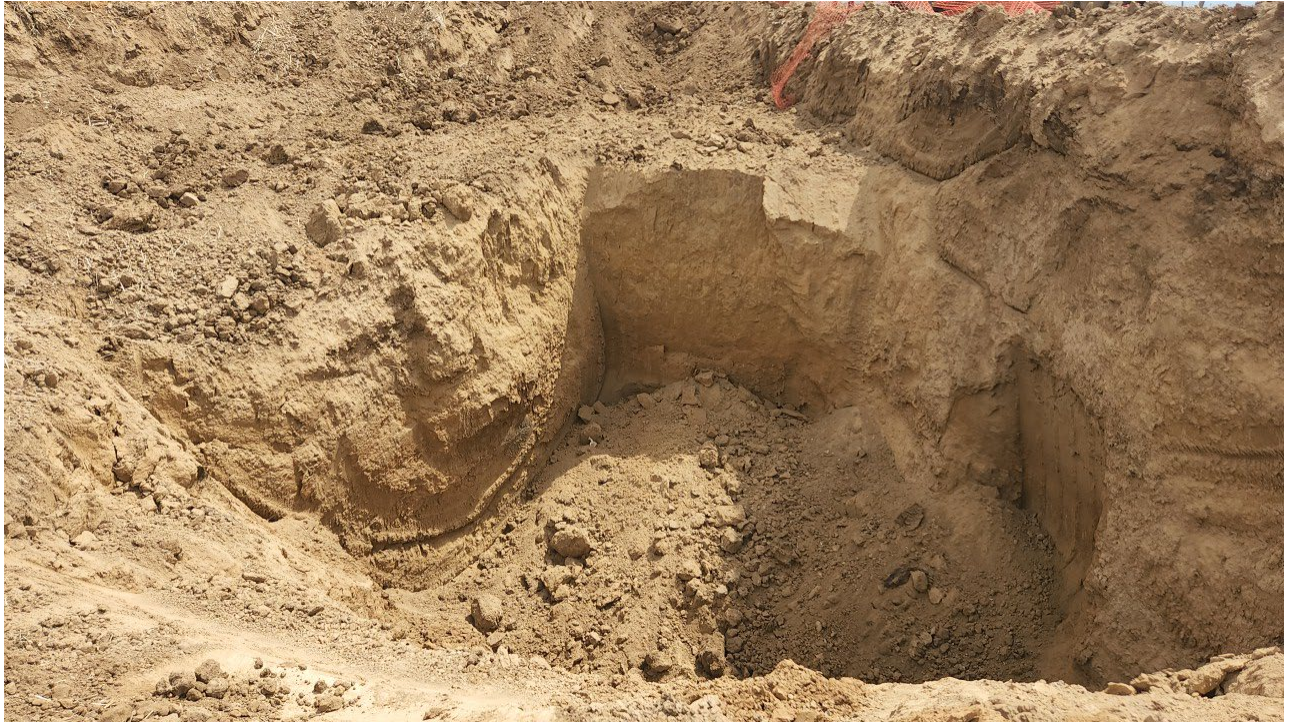
#5A – Champlin 67F – Inner Petroleum Exceedance Excavation – Former Produced Water Pit – Southern Sidewall of Excavation – S01@12.0' – PID 0.0ppm – Sample Submitted for Lab Analysis
