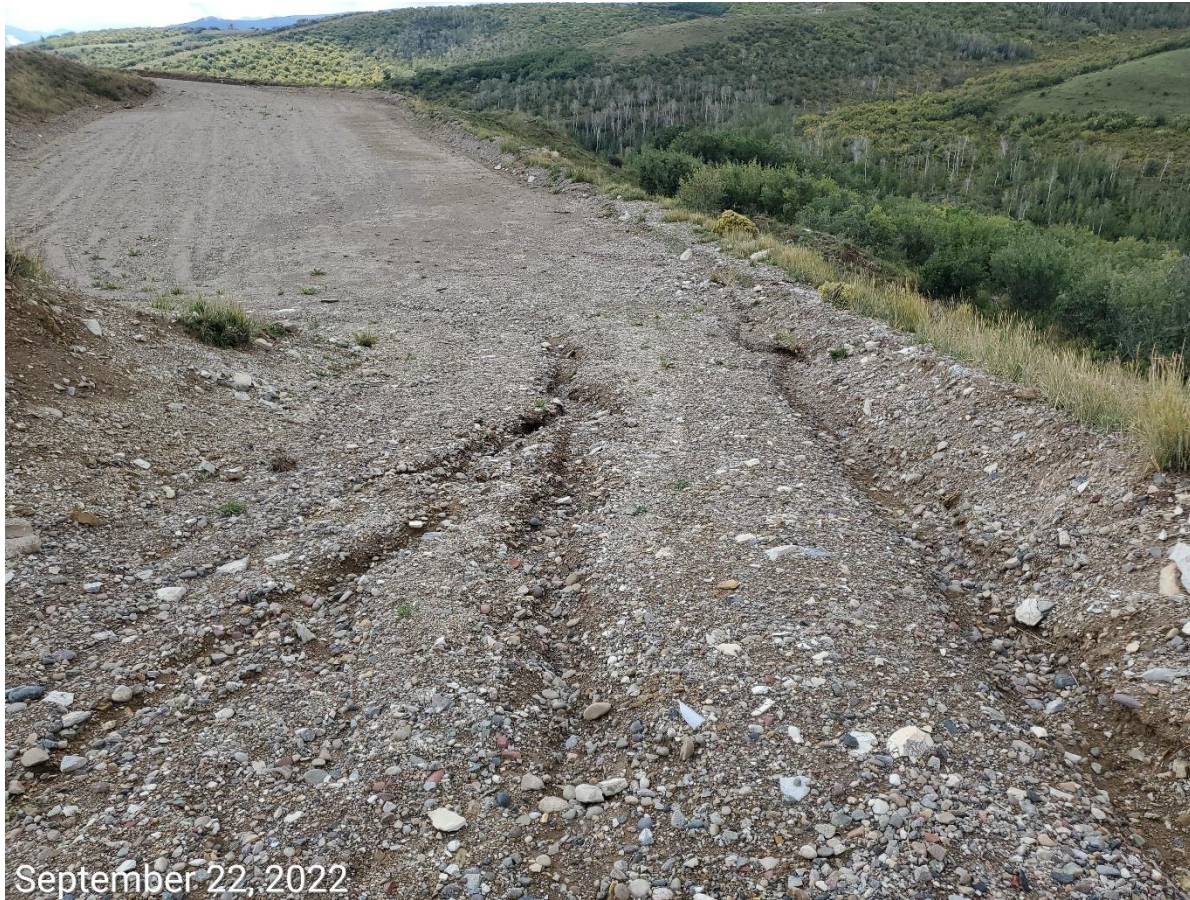
Photo 3: Photo taken from the former UIC facility site on the Location. Photo shows erosion degradation occurring along areas of the road leading to the former facility.
