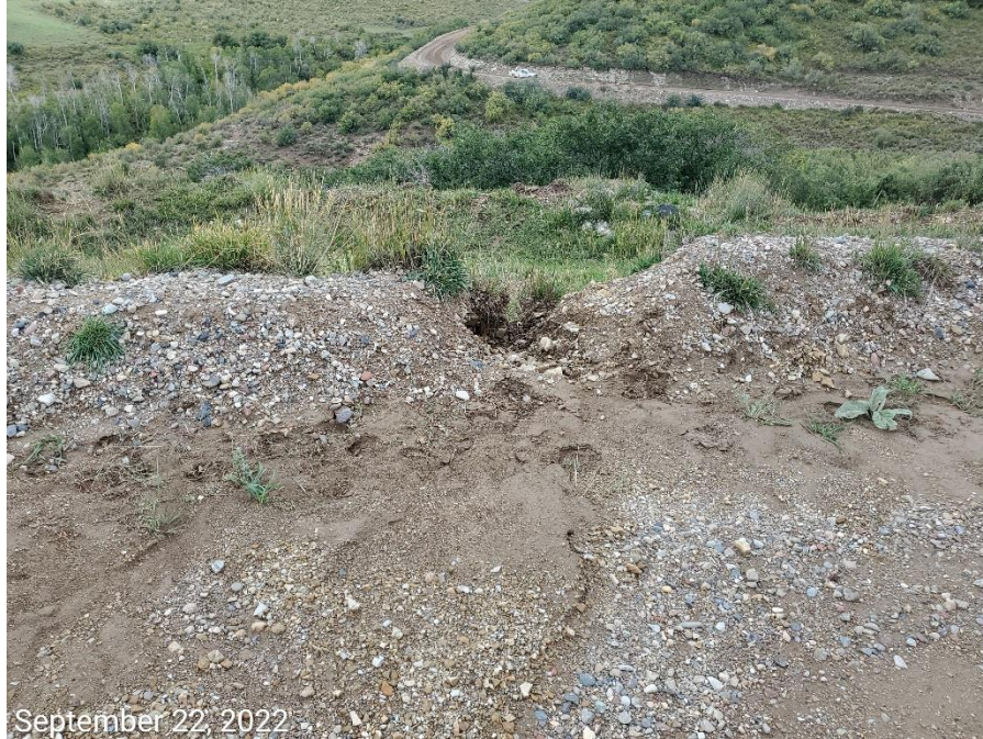
Photo 1: Photos taken from the sediment trap on the west end of the Location. Photos show stormwater runoff has resulting in gully degradation at the inlet. Hard hat in left photo used for reference.
