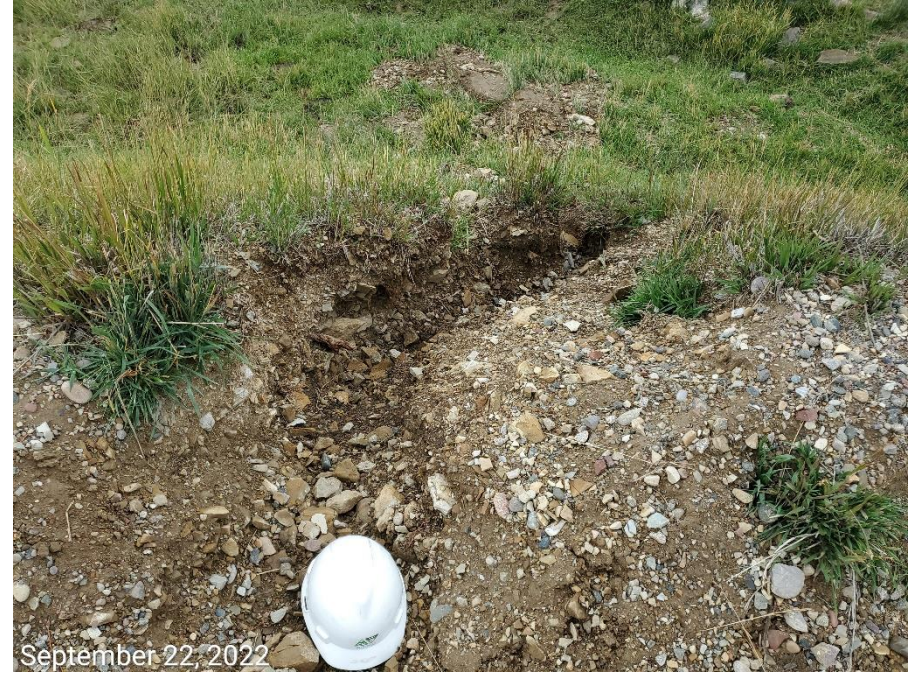
Photo 1: Photos taken from the sediment trap on the west end of the Location. Photos show stormwater runoff has resulting in gully degradation at the inlet. Hard hat in left photo used for reference.
