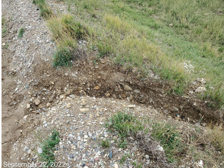
Photo 2: Continued from photo 1. Photo shows erosion degradation at the sediment trap.
