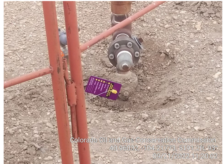
Photo 6 – Flowline Valve Tagged Out
