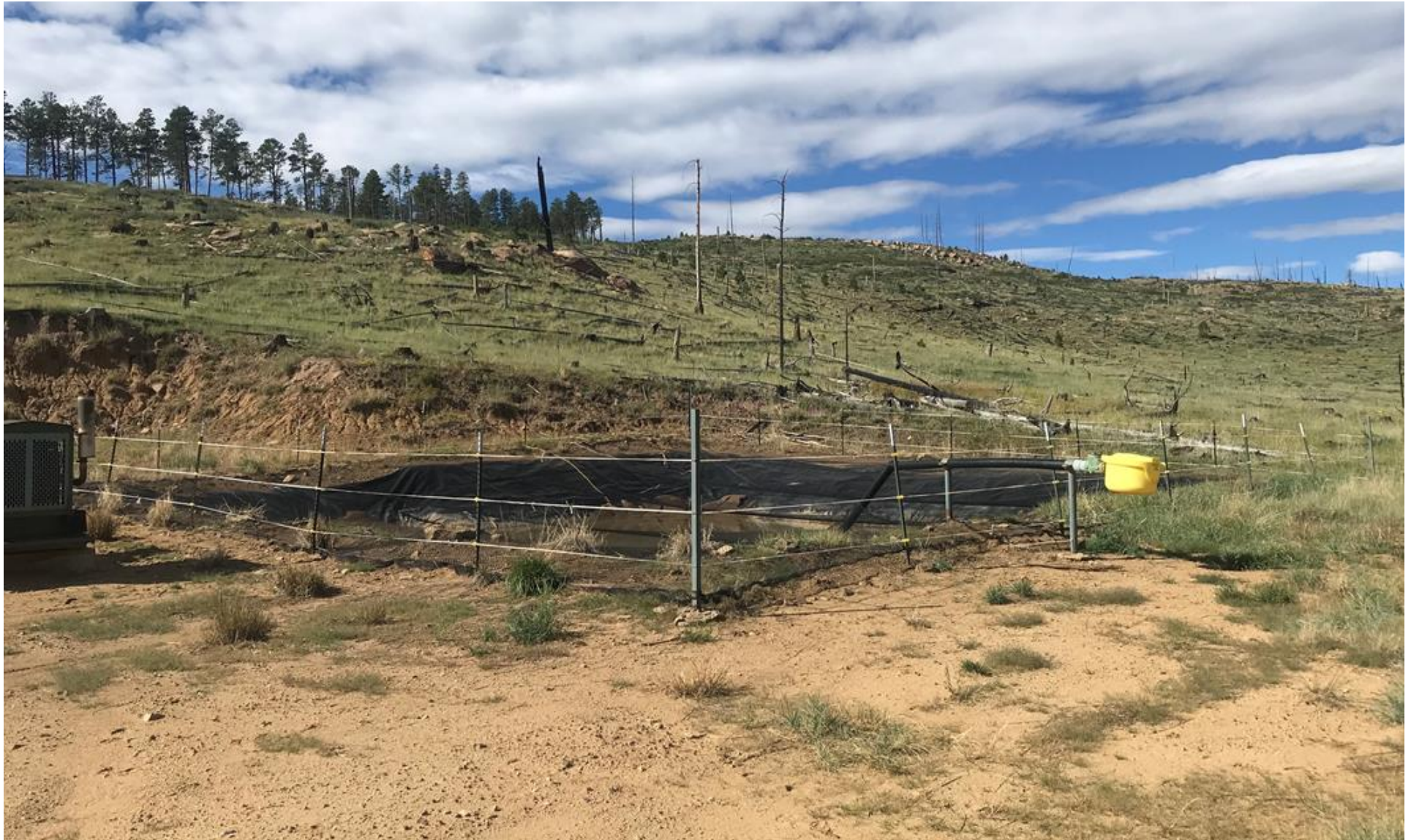
PHOTO 1: THE FENCING AROUND THE PRODUCTION WATER PIT HAS BEEN REPAIRED TO COMPLY WITH THE FENCING REQUIREMENTS PER THE 1002A RULES.
