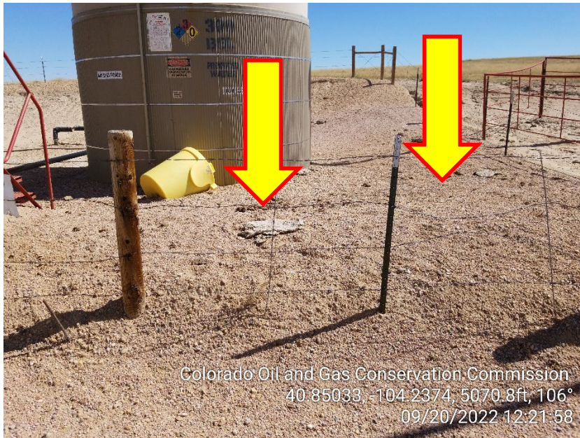
Photo 5 – Berm has been compromised by Livestock
