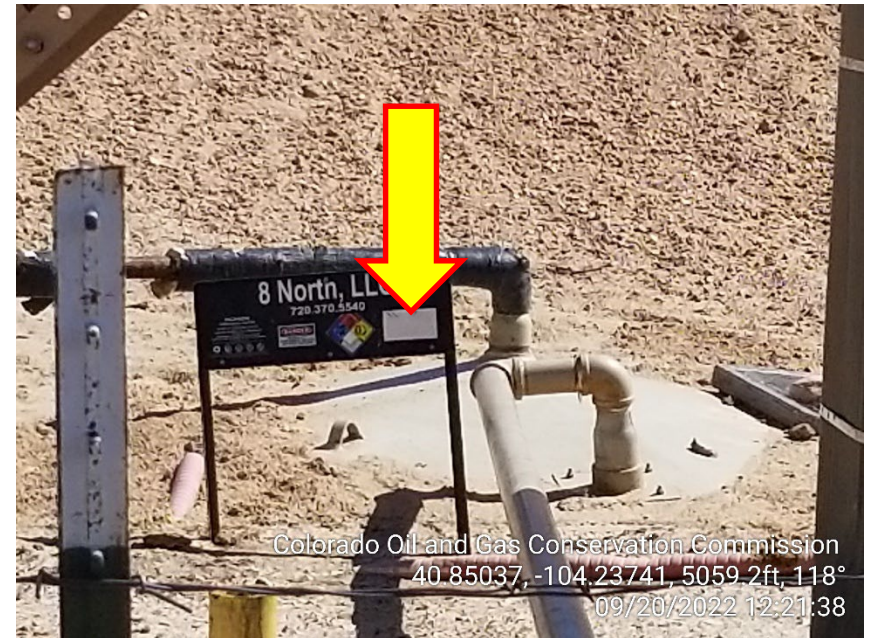
Photo 4 – Missing Capacity Label
