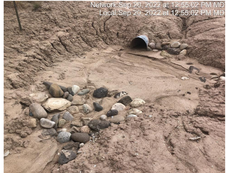
Photo #7762 Sediment trap is full run off of location is not being controlled.
