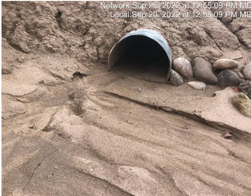
Photo #7763 Culvert capacity has been reduced due to Sediment migration.
