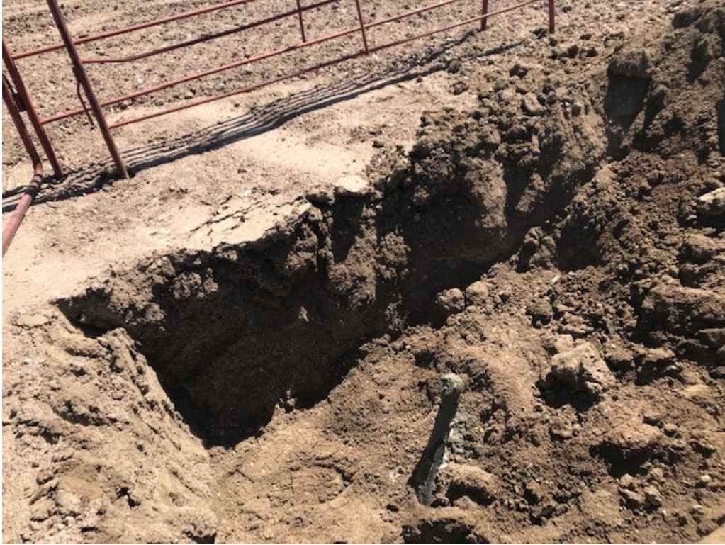
#9- Former Flowline at Wellhead Now Plugged with Cement
