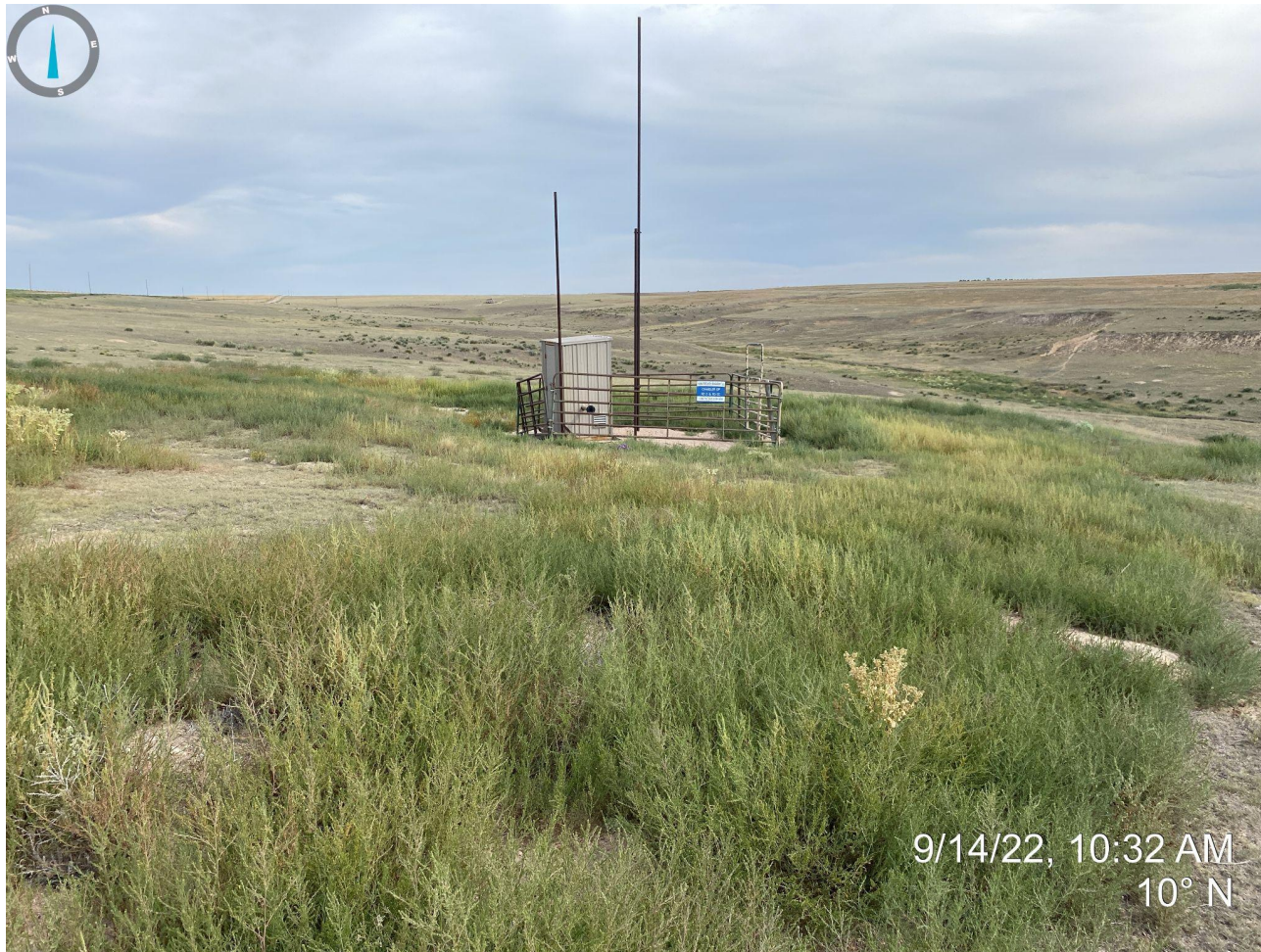
Photo 3. Taken south of location, facing north. Photo illustrates access road and location have not been reclaimed with presence of annual weedy vegetation, access road and location which have not been contoured, regraded, or revegetated. Oil and gas equipment remain on location.
