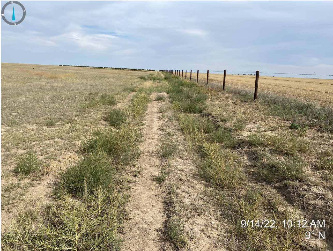
Photo 2. Access road facing north. Photo illustrates road has not been contoured or regraded; heavy rutting and annual weedy vegetation observed.
