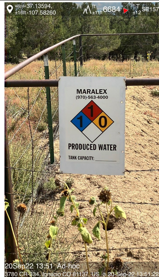
IMG 04 Tank capacity is not labeled
