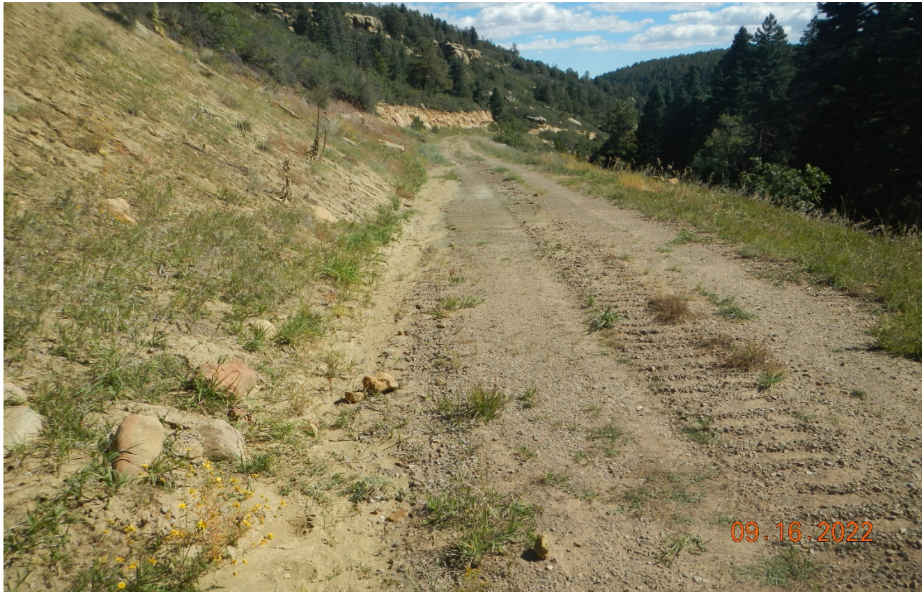
Photo 3. Facing northeast along the access road. The road is not recontoured. Fallen rocks have been moved off the roadway since previous inspection.
