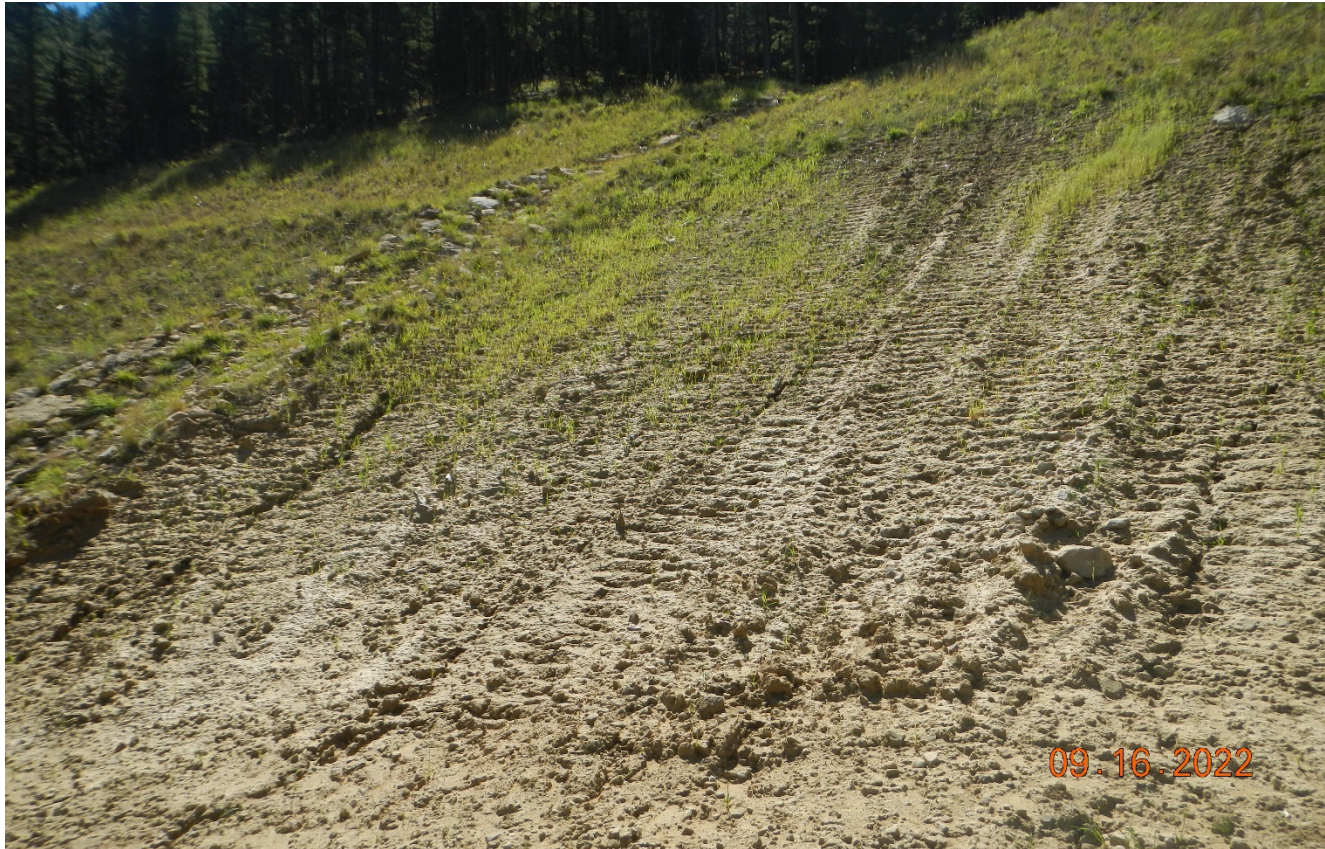
Photo 6. A portion of the location was regraded and dozer track. Additional BMP's (e.g. wattles) may be needed as there are some signs of erosion beginning to occur.
