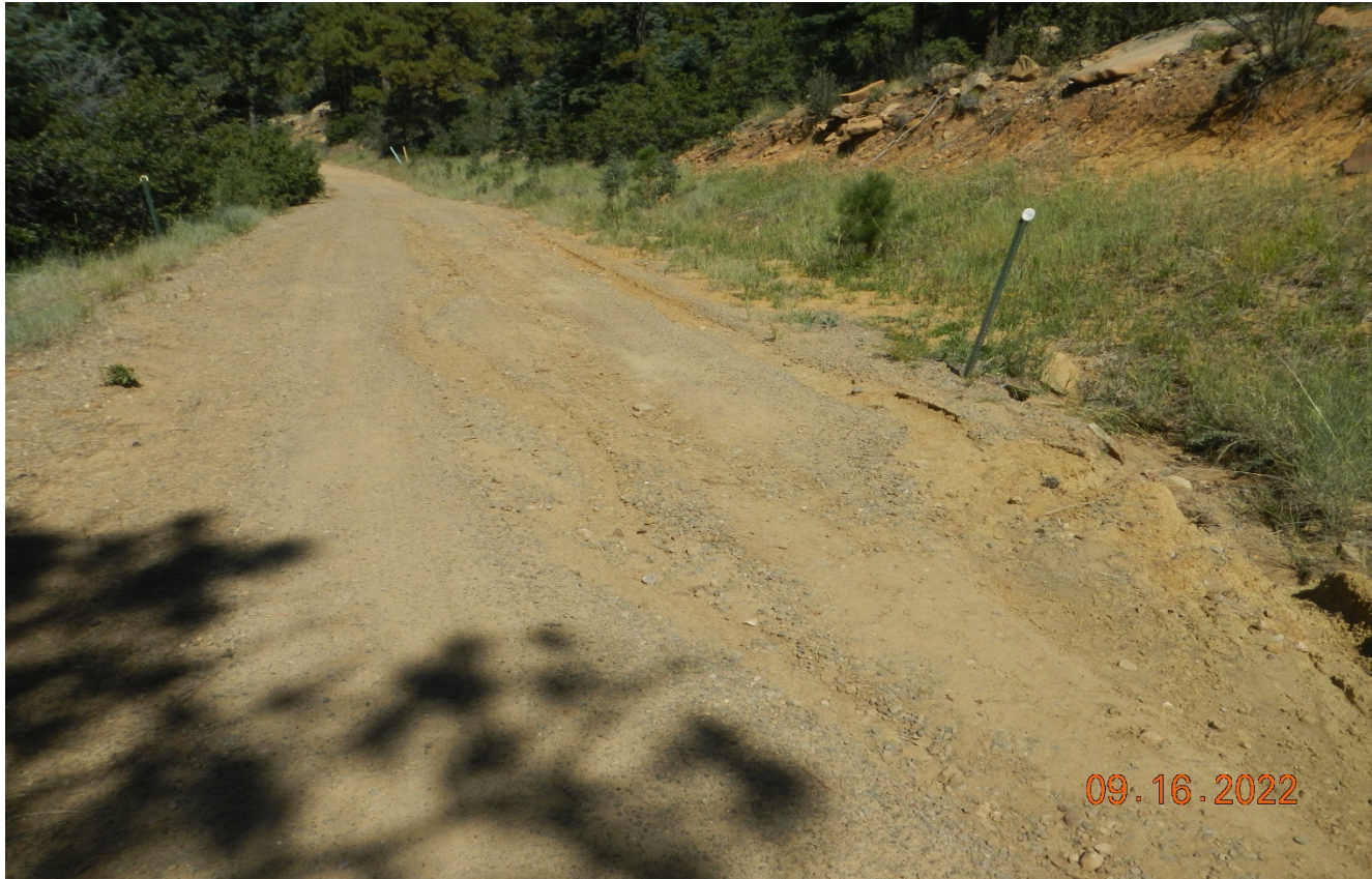
Photo 1. Facing southwest along the access road. Stormwater is bypassing the culvert causing erosion down the road. Lat/Long:37.28091,-104.90745
