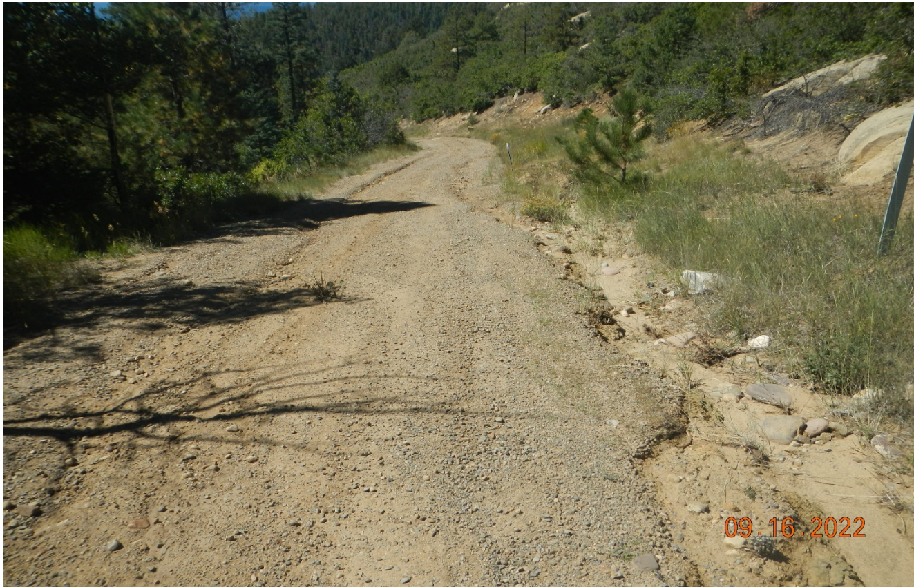
Photo 2. Further down the road. There is erosion along the road side that needs to be repaired and stabilized.
