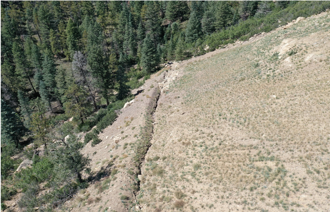
Photo 3. Facing west down at the location. A large berm was installed at the bottom of the location. There appears to be deep erosion into the berm where rock was not installed. BMP's such as rock check dams may be need to prevent accelerated erosion.
