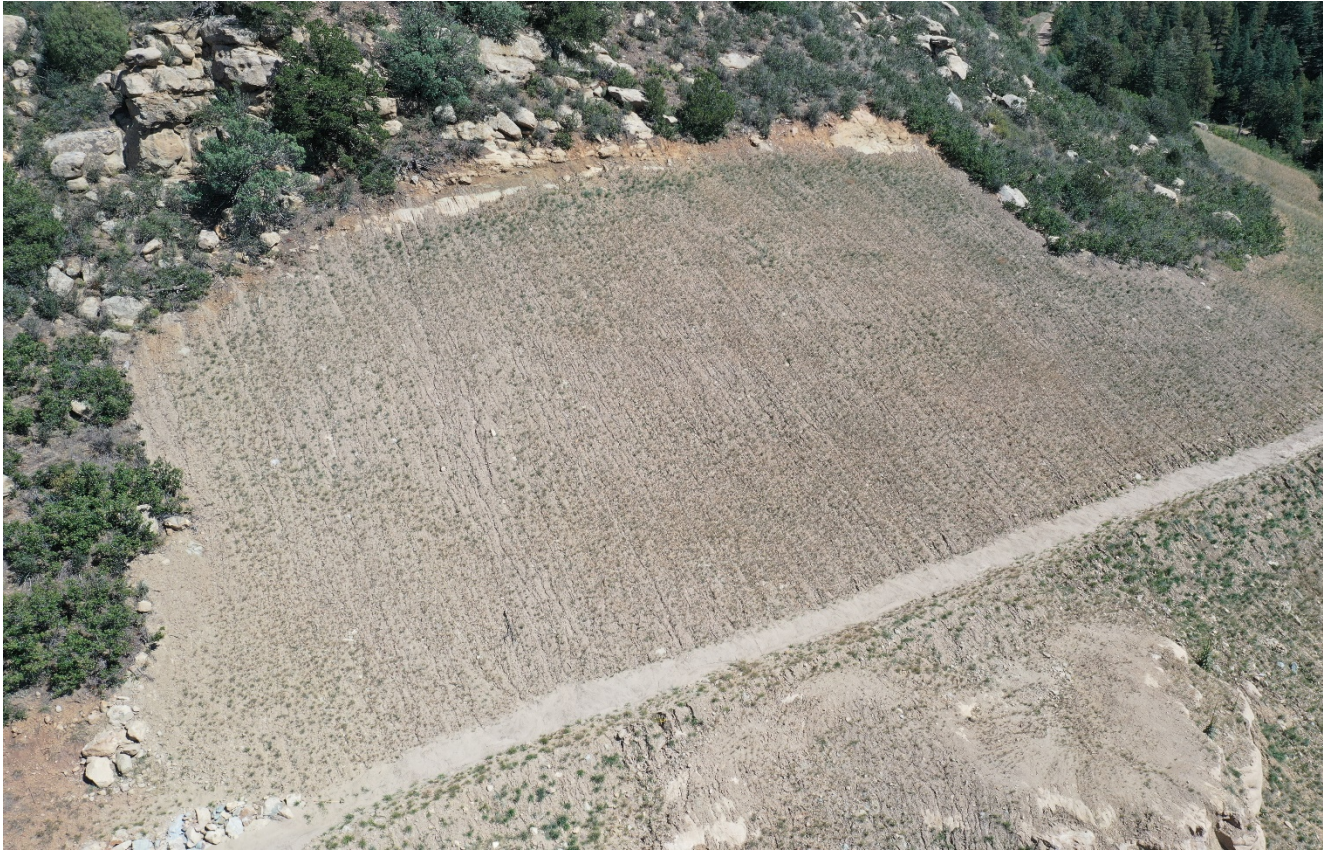
Photo 5. Facing toward the upper portion of the location. There is vegetation beginning to establish however additional BMP's may need to be installed.
