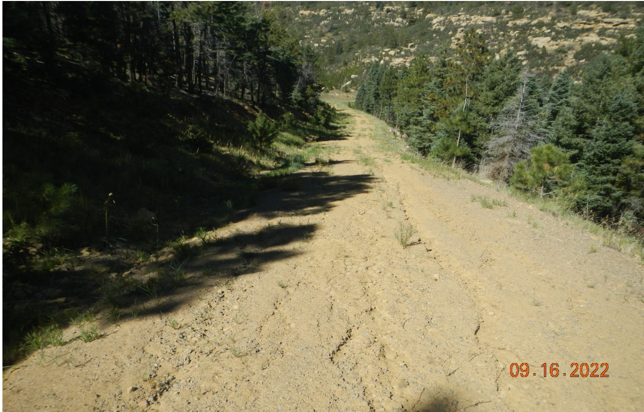
Photo 4. Facing northwest toward road turns down the hill side into the canyon. There is some initial signs of erosion down the road which may require additional BMP's such as a water bar.
