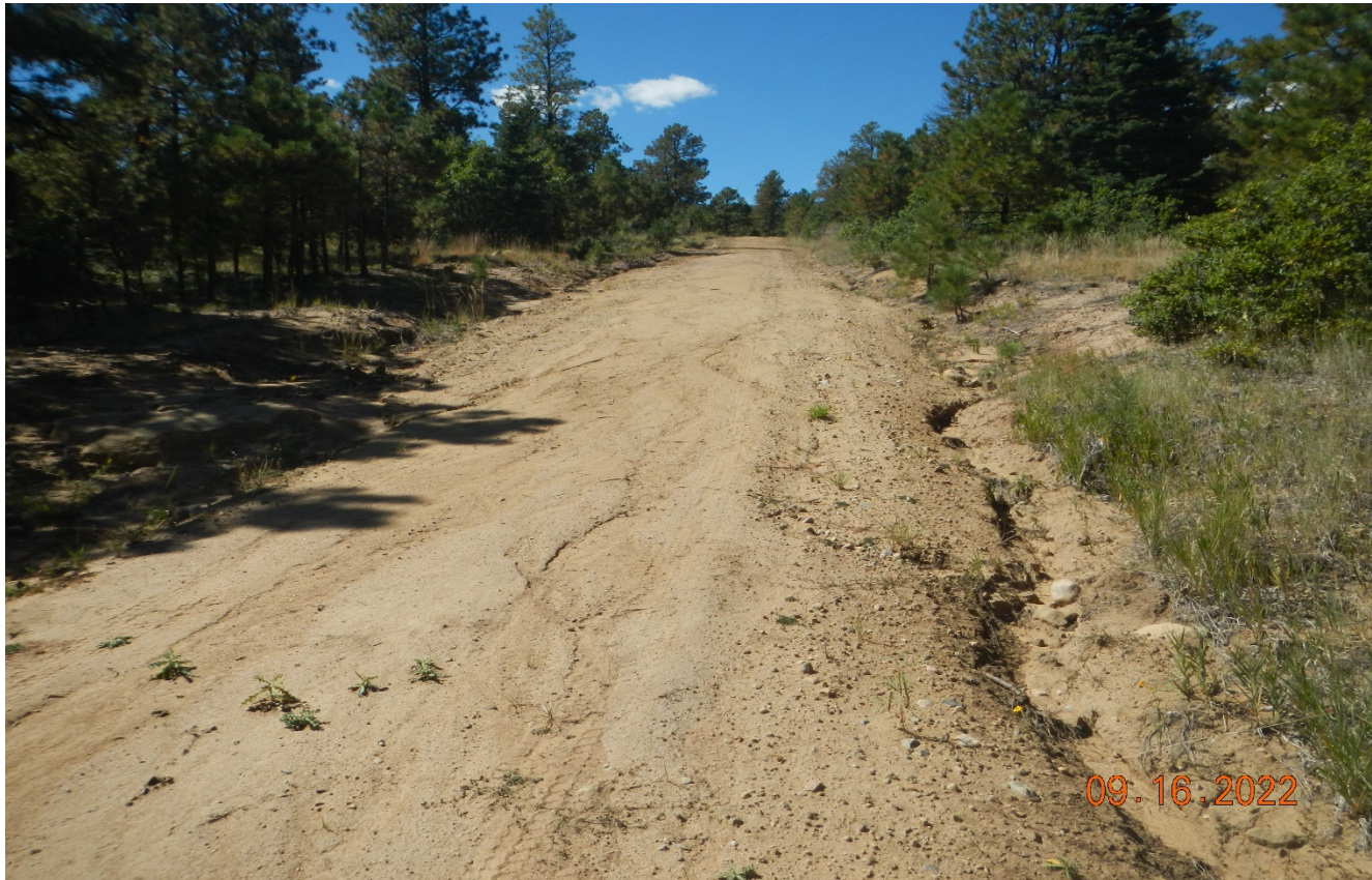
Photo 3. Facing back to the south west. There is erosion beginning to occur along the roadsides and additional BMP's are needed in this area.
