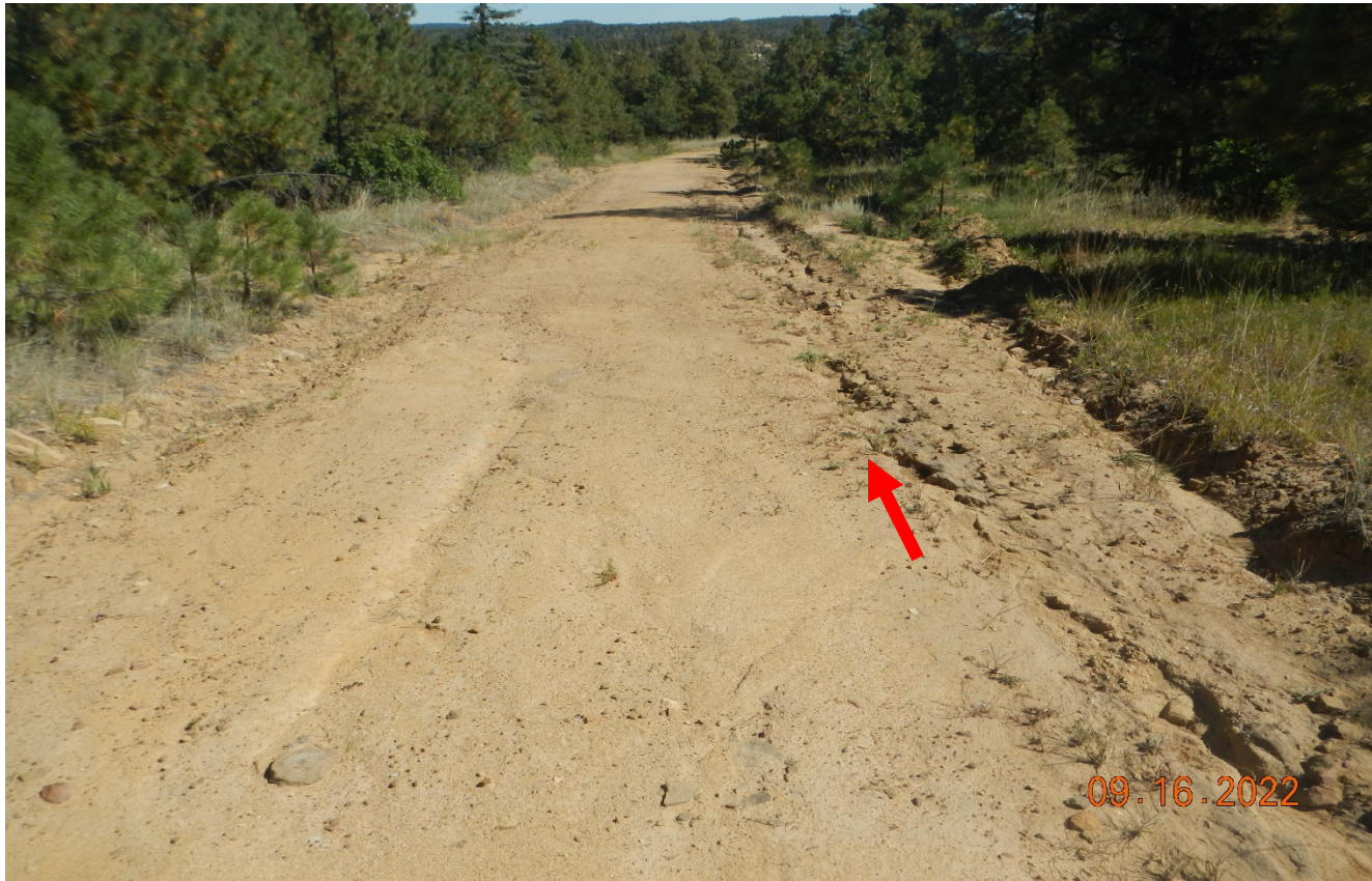
Photo 2. This area of the road needs additional work due to signs of stormwater flowing past the diversion ditch on the right which is beginning to create erosion down the road.
