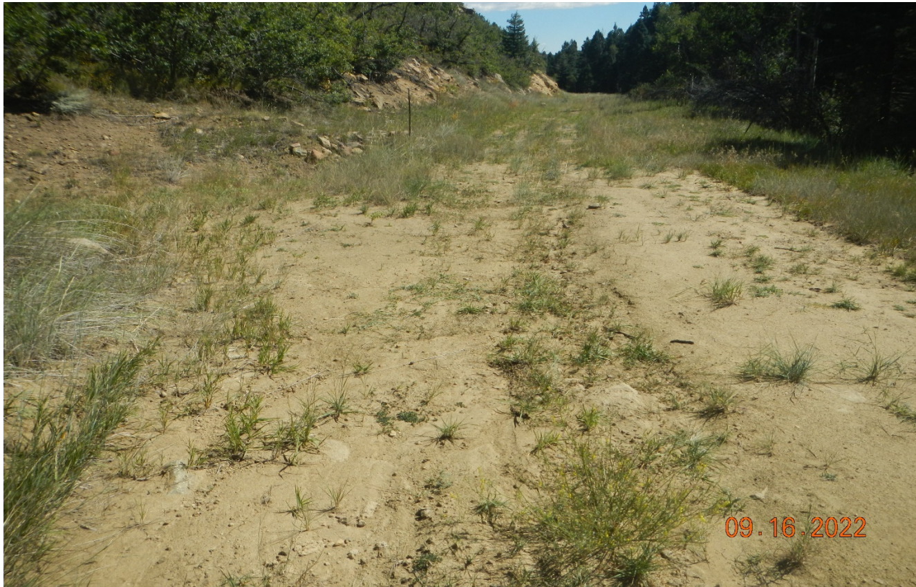
Photo 6. Facing east along the access road. This area may need some hand work to get stormwater better directed toward the culvert.
