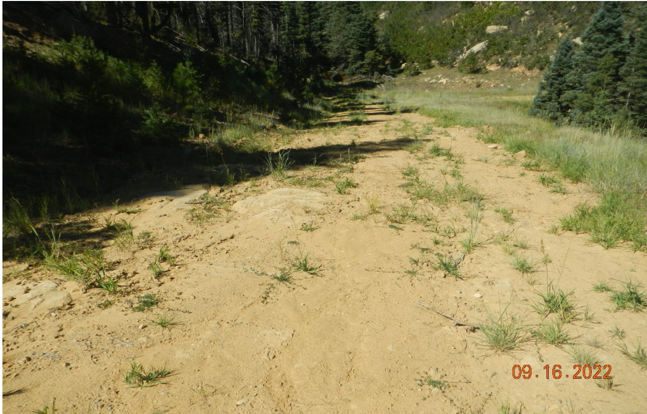
Photo 5. The road was graded down to the canyon bottom and erosion was repaired. This area has a long stretch without culverts and may require additional stabilization or vegetation establishment. This area was previously observed to be eroded.
