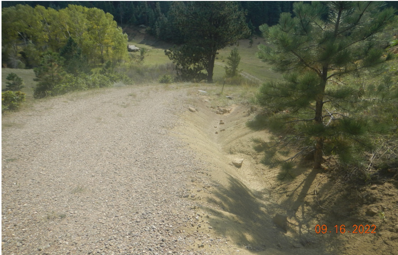
Photo 2. Facing back down the road. There is erosion along the road side that needs to be repaired and stabilized.
