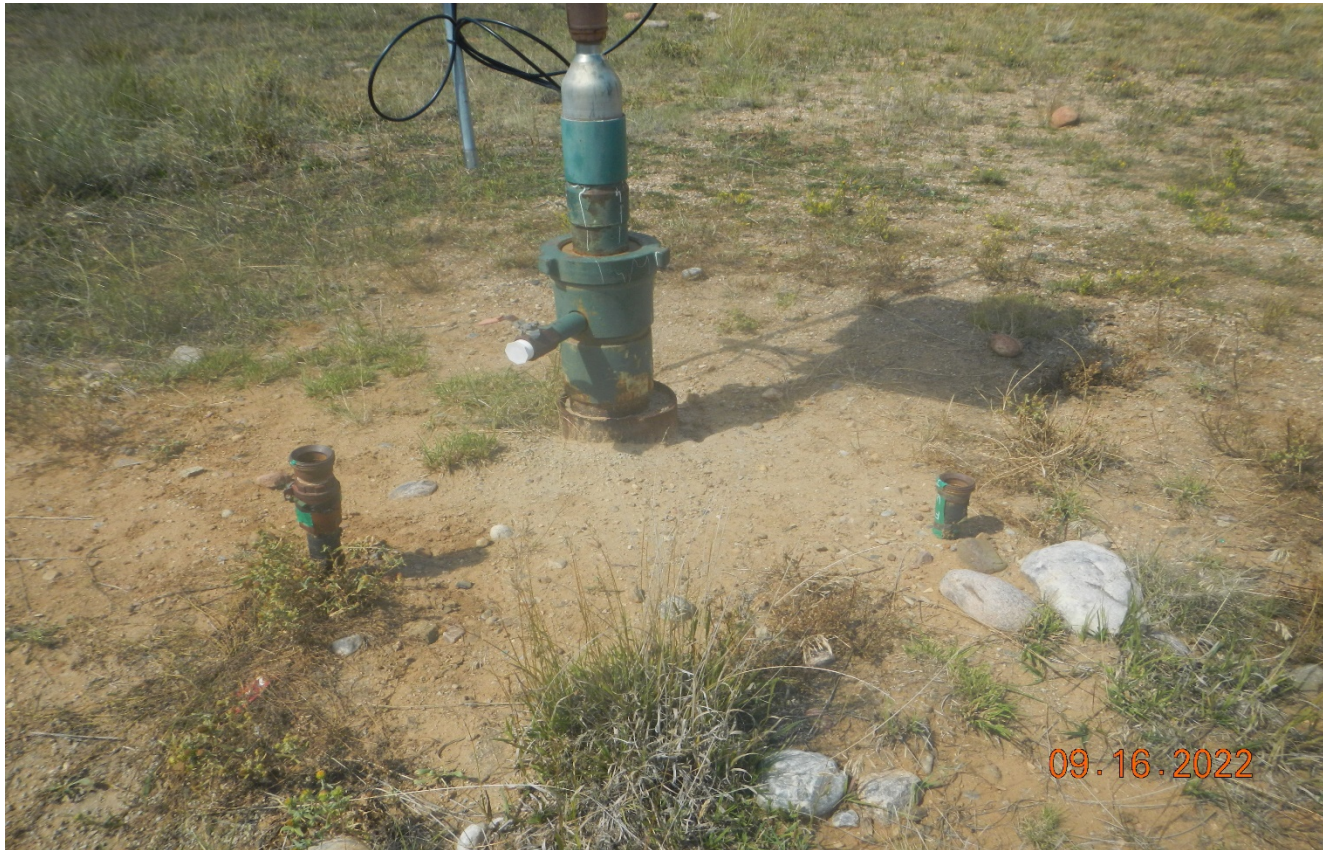
Photo 5. There are 3 pipe risers with no OOSLAT.
