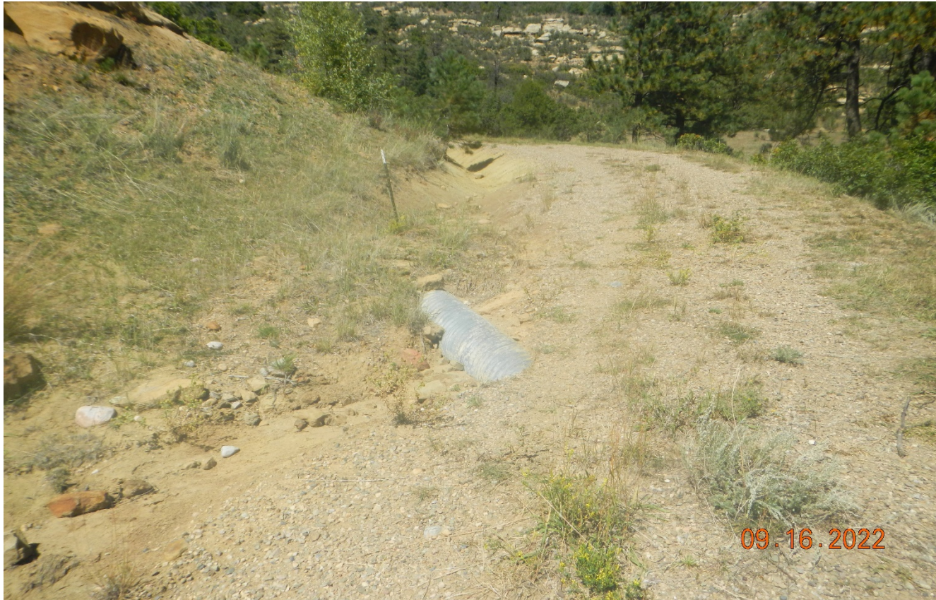
Photo 1. Facing north along the access road. Stormwater is bypassing the culvert causing erosion down the road.
