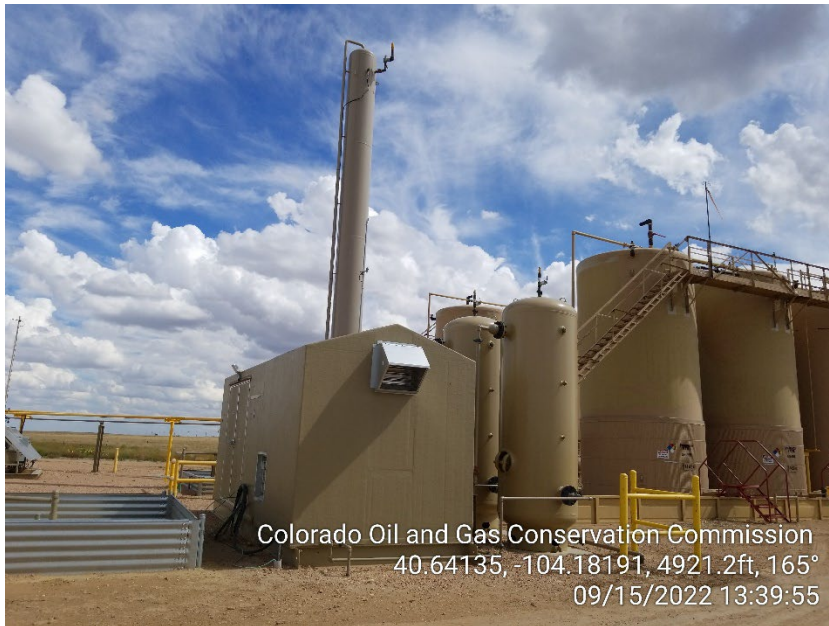
Photo 11 – VRT, Air Unit, Tanks
