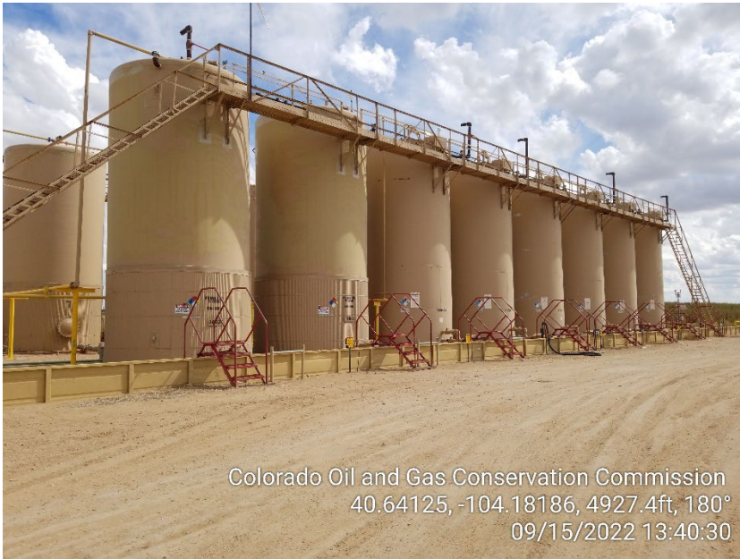
Photo 13 – Tank Battery
