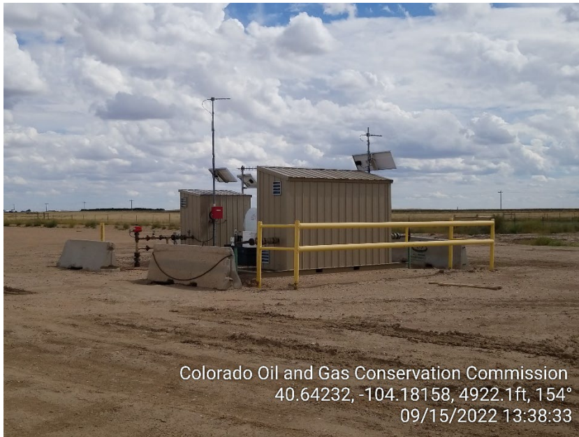
Photo 7 – Gas Lift Injection Meter Houses
